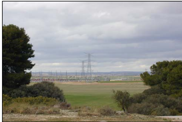
Figure 2.2: Example of a substation set in a rural location surrounded by crop fields.
