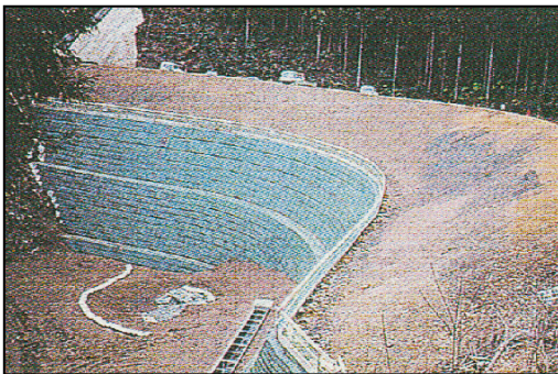
(a) Under construction
