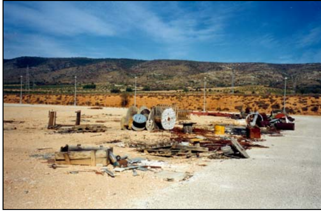
Figure2.5: Substation lacking waste storage area.
