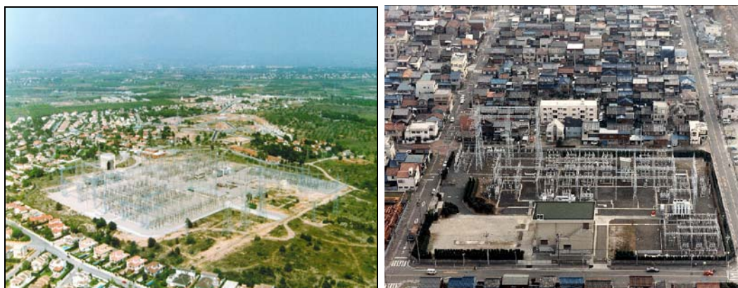
Figure 2.1: Substation surrounded by densely populated area.
