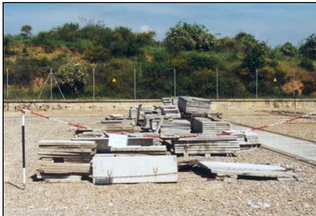
Figure 2.6: The area for storing the concrete covers of the cable troughs has been clearly demarcated by a chain-link fence and a sign.
