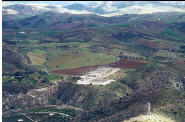
Figure 2.9: Poor choice of gravel colour has made the visual impact of this substation much greater.
