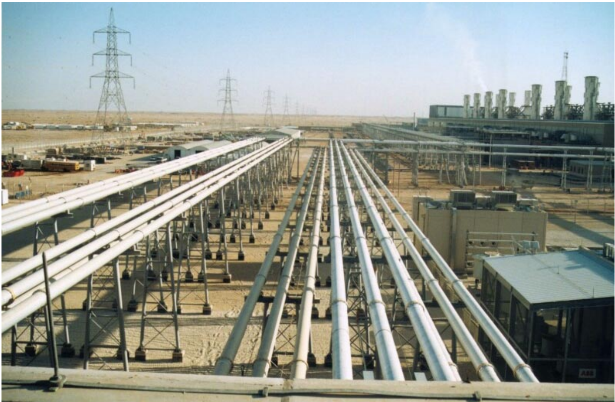
Figure 15: Views of the 420 kV PP9 GIL: erection and layout.
