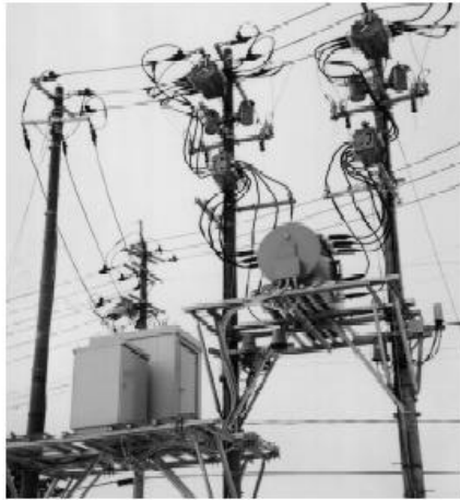
Figure A 23: Driven-arc type fault current limiter
