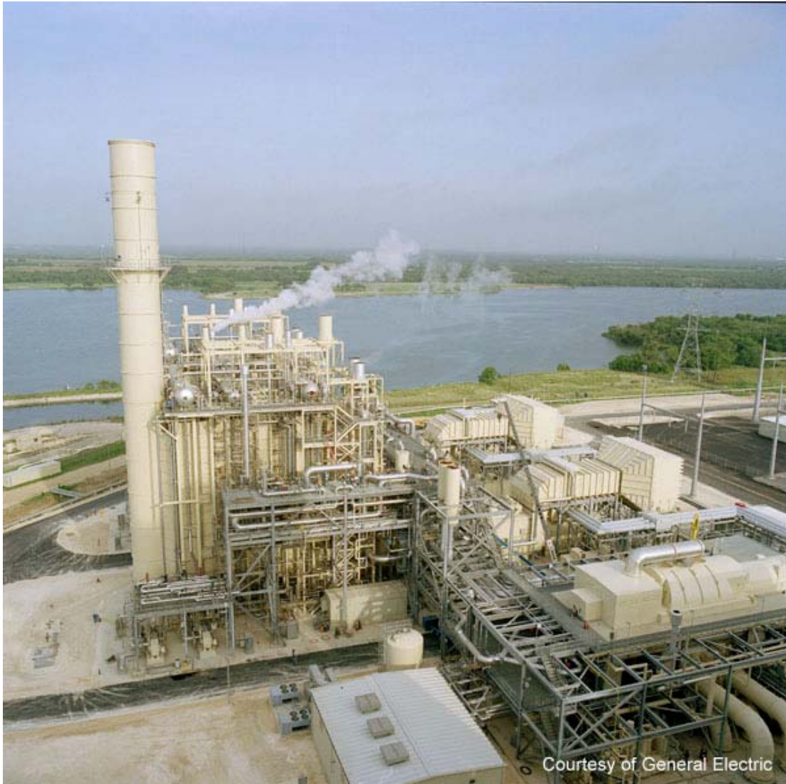
Figure 2-16: A multi-shaft combined-cycle power plant showing two gas turbines, a steam turbine and HRSGs (Source: GE Power Systems)
