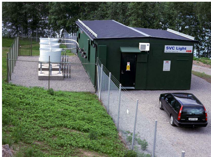
Figure 6.5 View of Hagfors installation showing the SVC Light equipment and the phase reactors.
