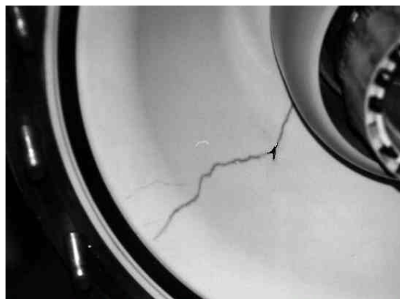
Figure 1.7 Particle induced breakdown on the surface of a 400kV GIS spacer. [4]
