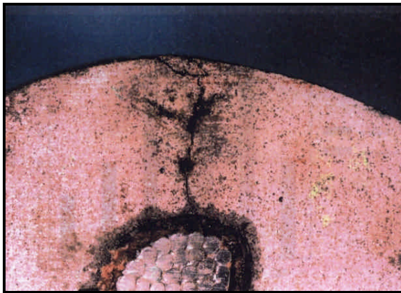
Figure 1.5 Aging process in a resin cable joint caused by partial discharges and treeing [2]
