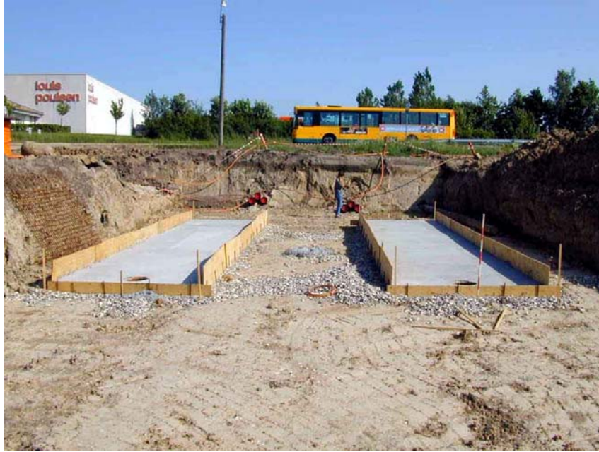
Figure 96: Foundations for direct buried 400 kV Joints
