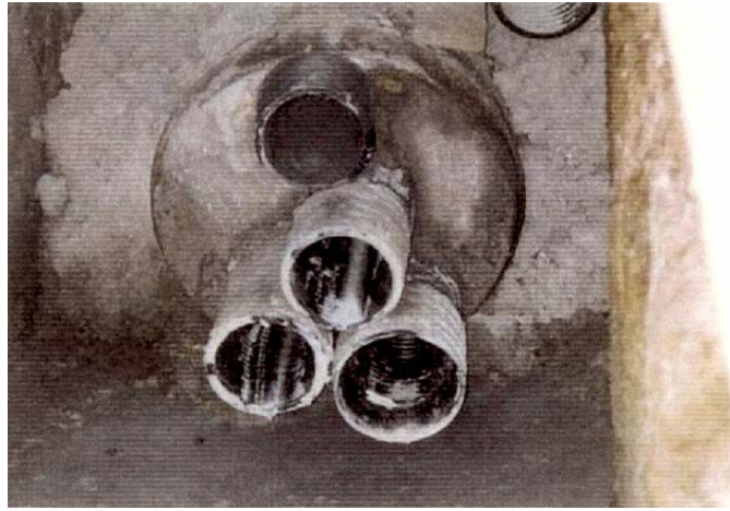
Figure 58: Example of ferromagnetic tubular shielding
