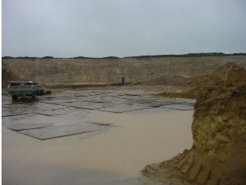
Figure 88: Excavation before construction of a 400 kV Transition Compound
