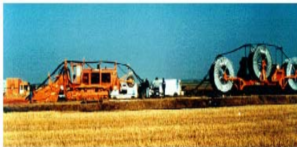
Figure 66: Mechanical laying (French site)
