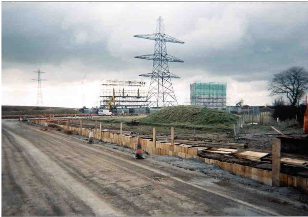
Figure 94: Temporary visual impact during the construction of a 400 kV Transition Compound
