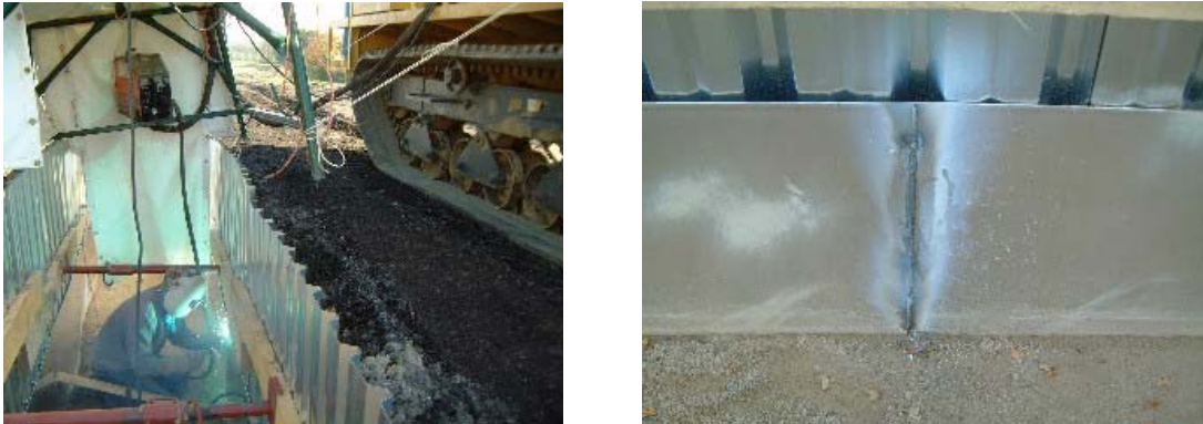
Figures 56a and 56b: Welding on site of aluminium sheets
