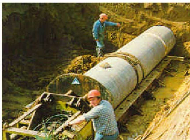
Figure 67: Pipe jacking (French site)
