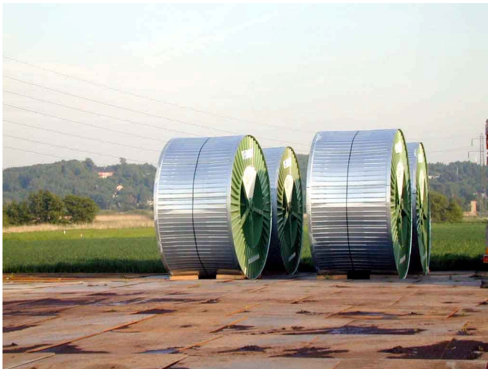
Figure 87: Storage area for drums with steel plates for soil protection
