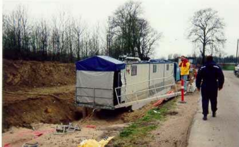
Figure 69: temporary enclosure for jointing
