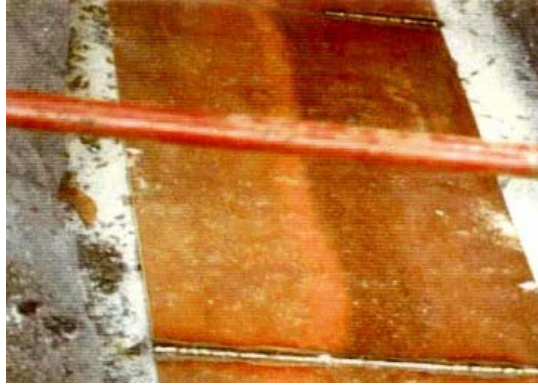
Figure 54: Example of shielding with copper sheets [30]
