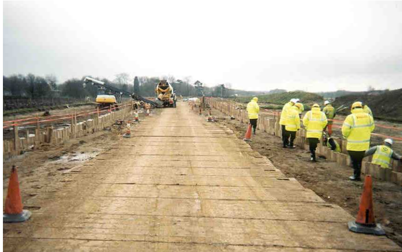
Figure 91: Provisional track during the construction of a 400 kV cable system
