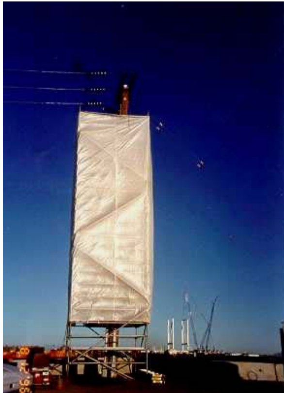
Figure 70: temporary enclosure for terminating
