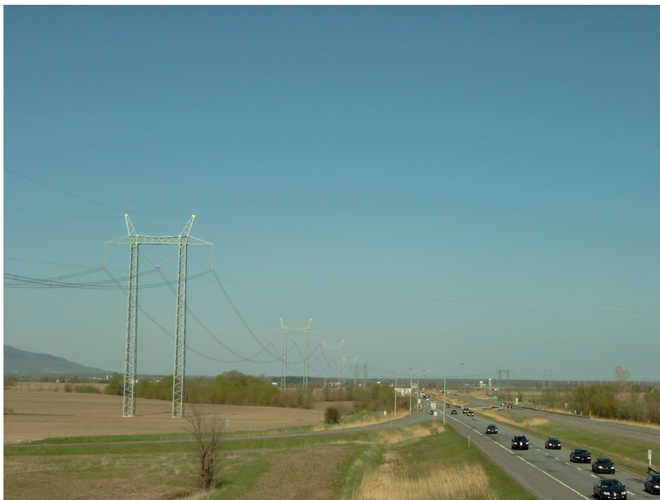
Figure 2: 735 kV Steel lattice H frame line parallel to highway
