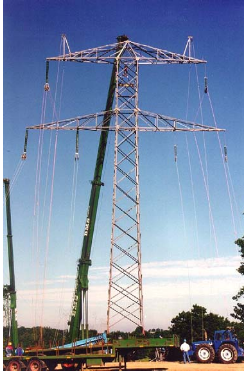
Figure 72: Erection of Danube tower with a 400 kV circuit and a 150 kV circuit.
