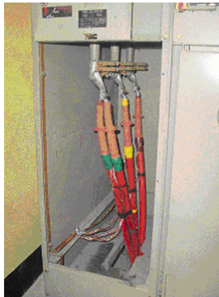
Modular cubicle with unipolar cables
