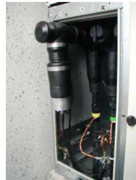
Figure 5-4 Capacitive coupling in gas insulated MV cells
