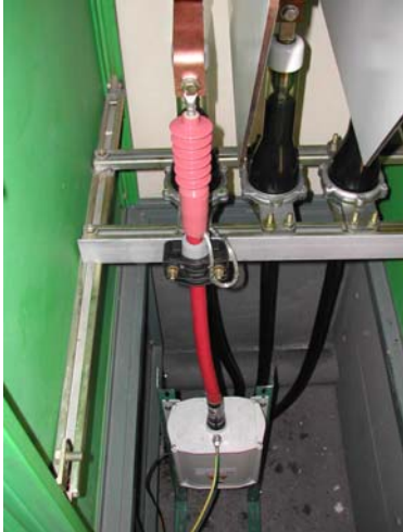
Figure 5-3 Capacitive coupling in air insulated MV cells
