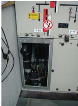
Figure 5-4 Capacitive coupling in gas insulated MV cells
