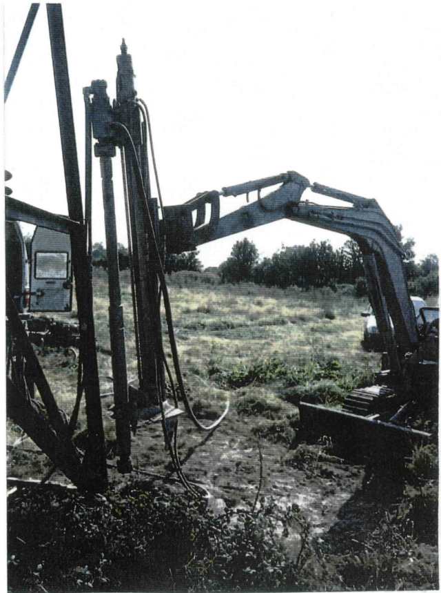
FRANCE (EDF) Grouted bored micropiles
