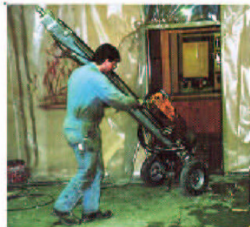
Self Drilling, Hollow Injection Grouted Micro Piles complying with DIN 4128, EAU E 28 and draft CEN/TC 288/WG 8 with ultimate loads from 220 kN to 3460 kN (50 to 778 Kips)
