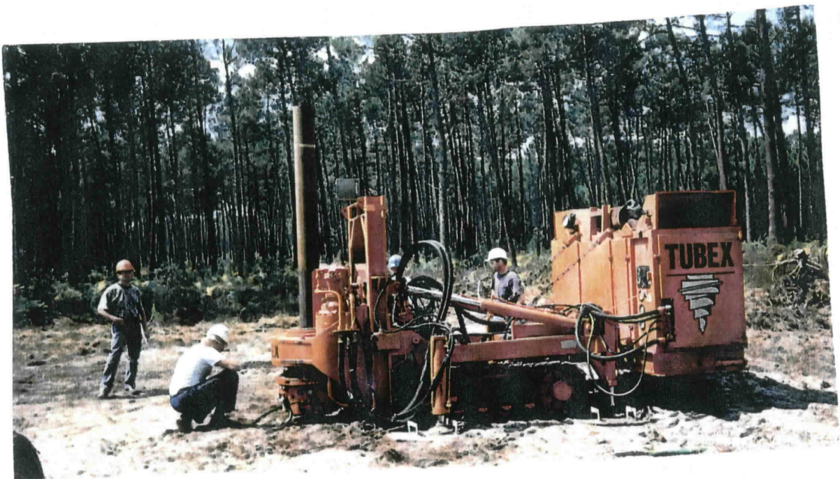
FRANCE (EDF) Screwed metallic piles
