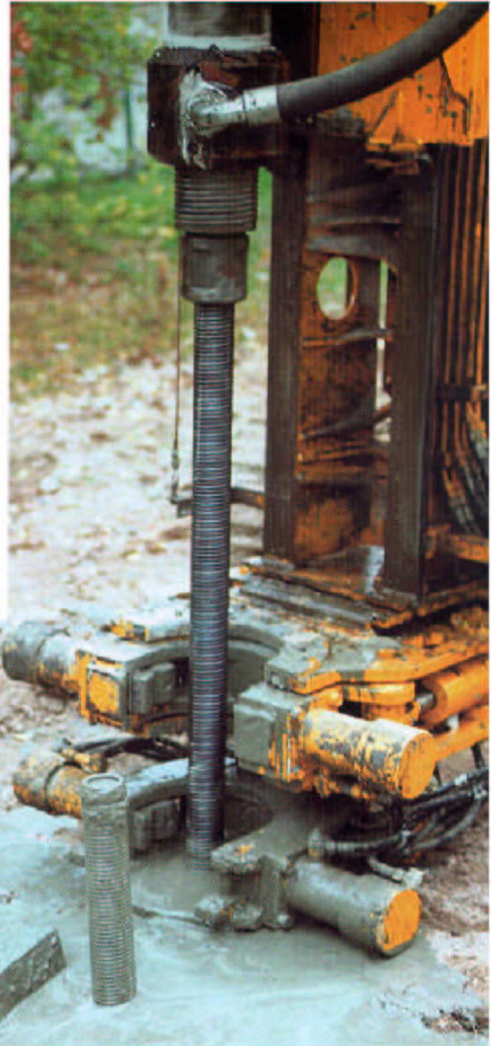
Self Drilling, Hollow Injection Grouted Micro Piles complying with DIN 4128, EAU E 28 and draft CEN/TC 288/WG 8 with ultimate loads from 220 kN to 3460 kN (50 to 778 Kips)
