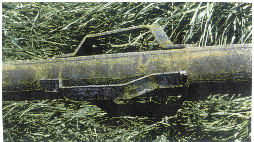
FRANCE (EDF) Grouted bored micropiles
