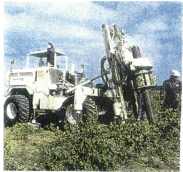
FRANCE (EDF) Screwed metallic piles
