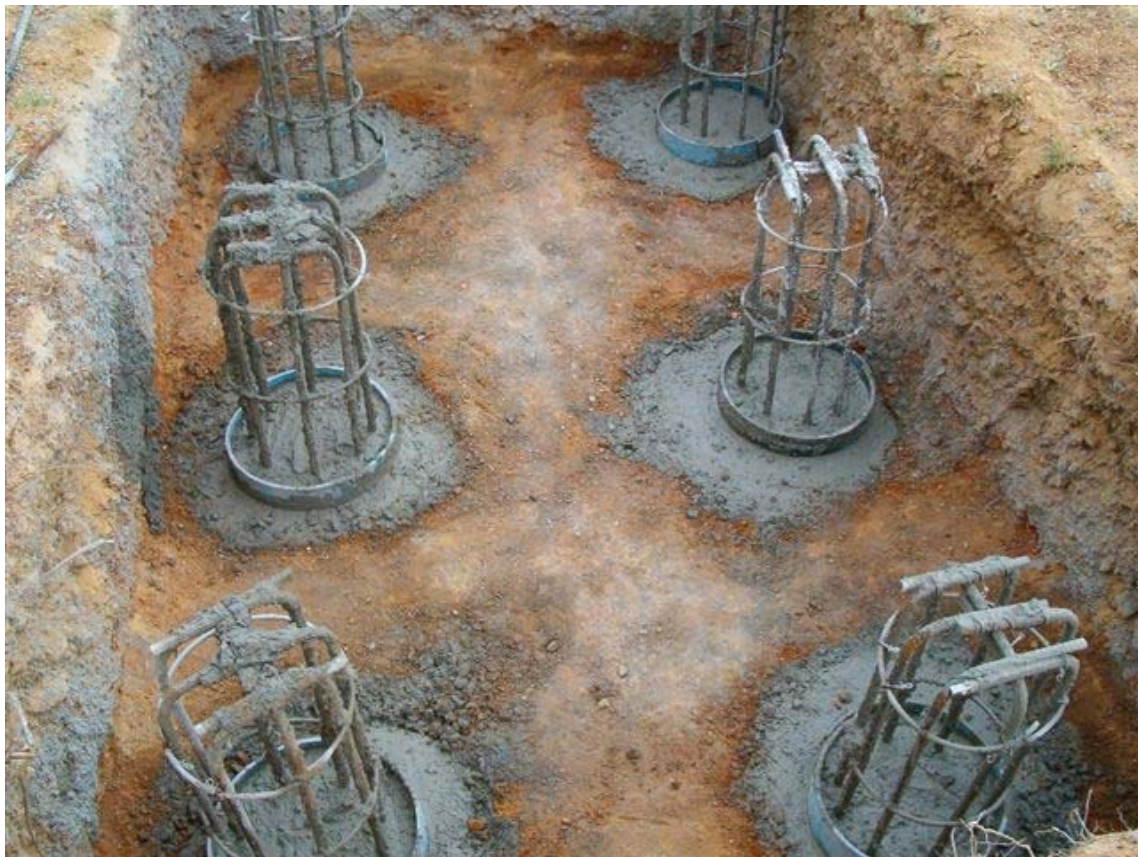
Figure 3A.7b – Auger-pile foundations after concreting of the individual auger-piles
