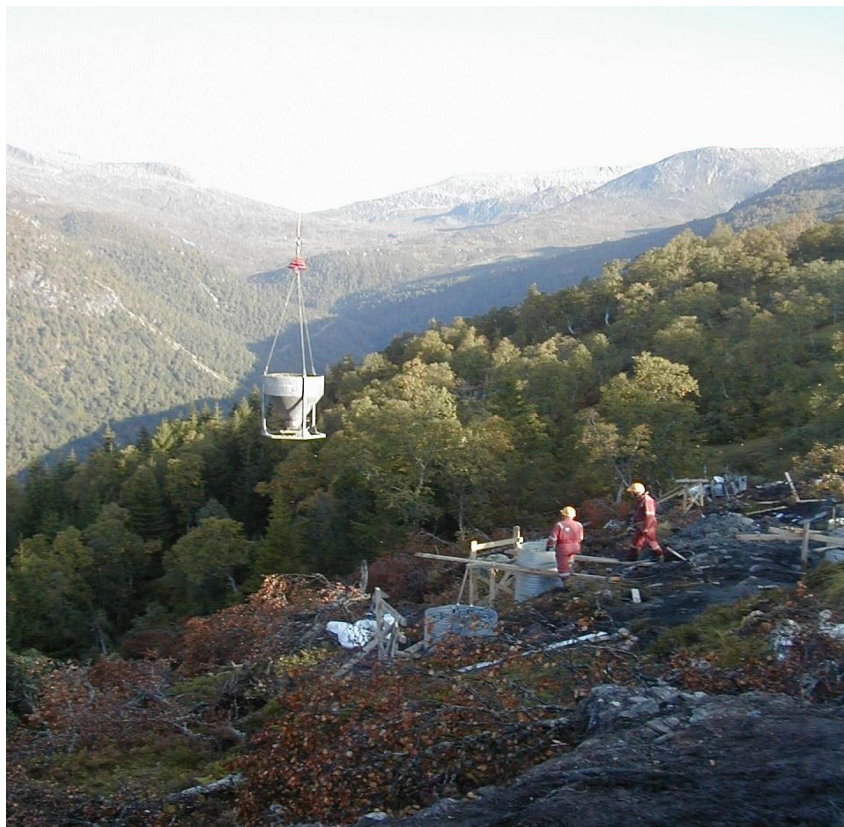
Figure 8.3 – Transportation of foundation concrete by helicopter
