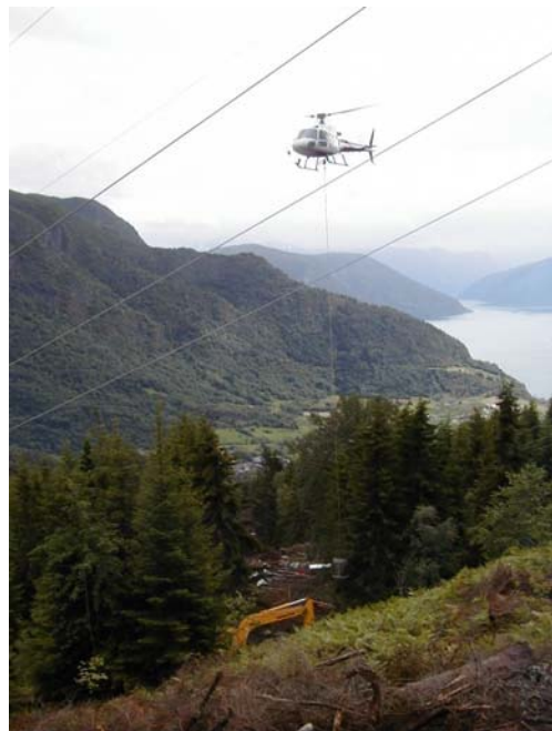
Figure 6.2 – Transportation of concrete by helicopter
