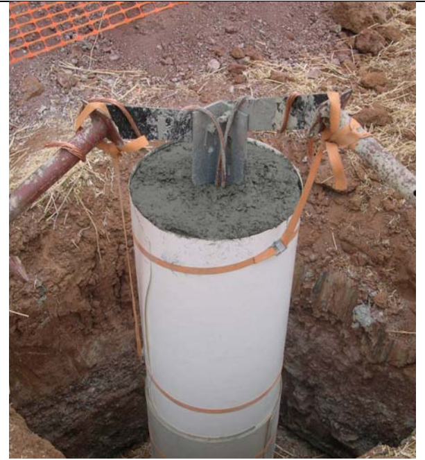
Figure 3.12 – Disposable formwork
