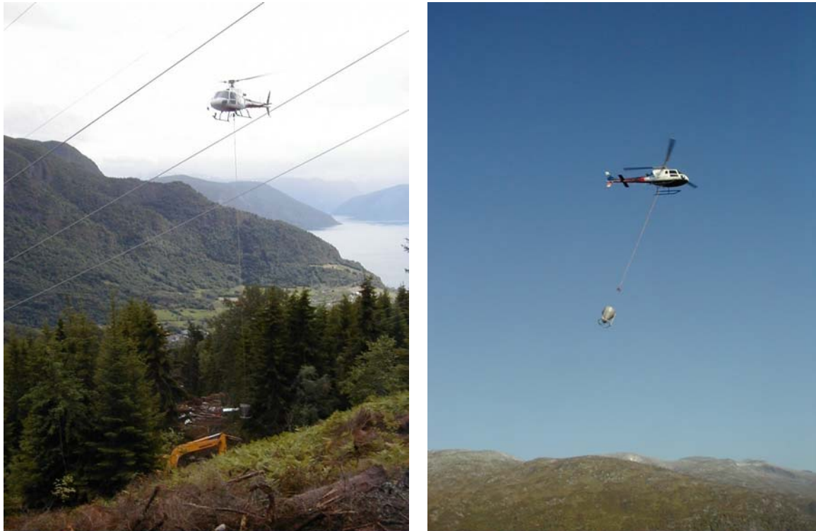
Figure 6.3 - Transportation of foundation concrete by helicopter
