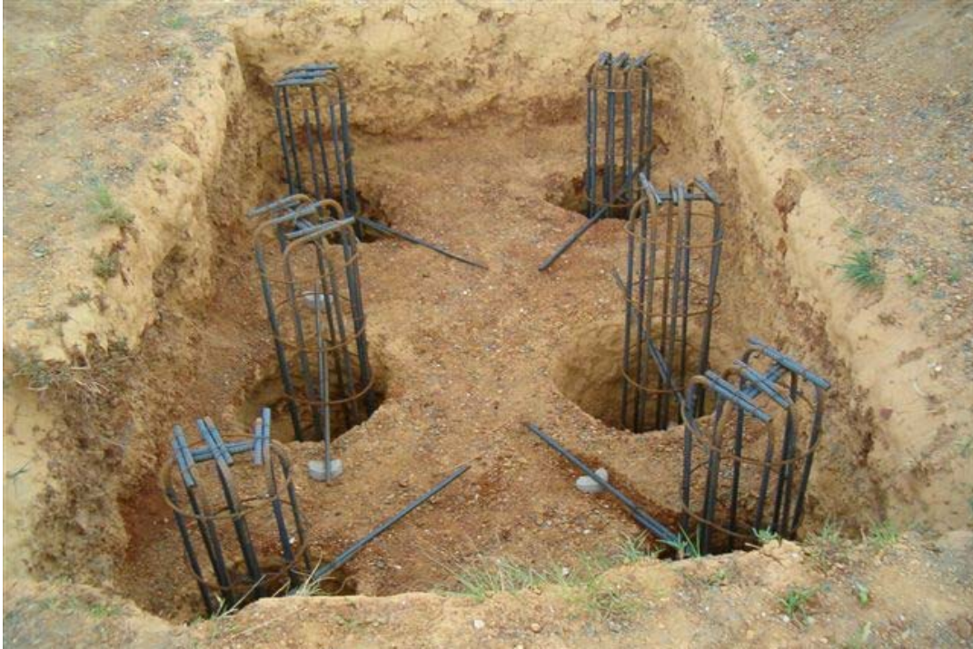
Figure 3A.7a – Auger-pile foundations before concreting of the individual auger-piles
