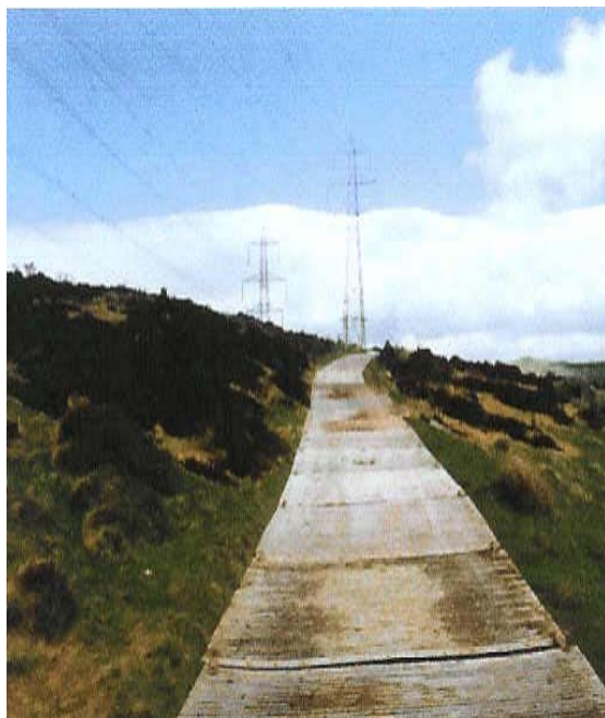
Figure 6.1 - Aluminium track way panels
