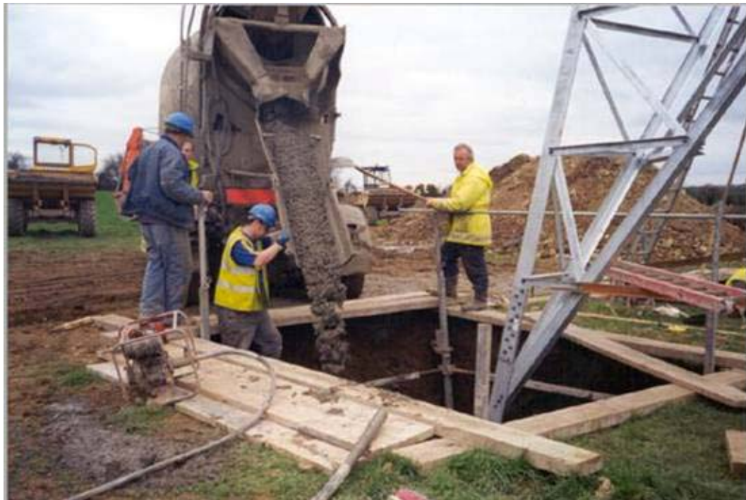
Figure 4.6 – Concrete placing
