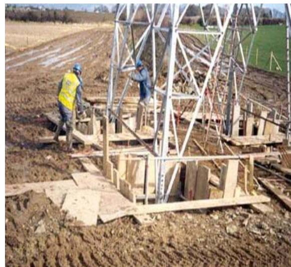
Figure 4 – Stub setting
