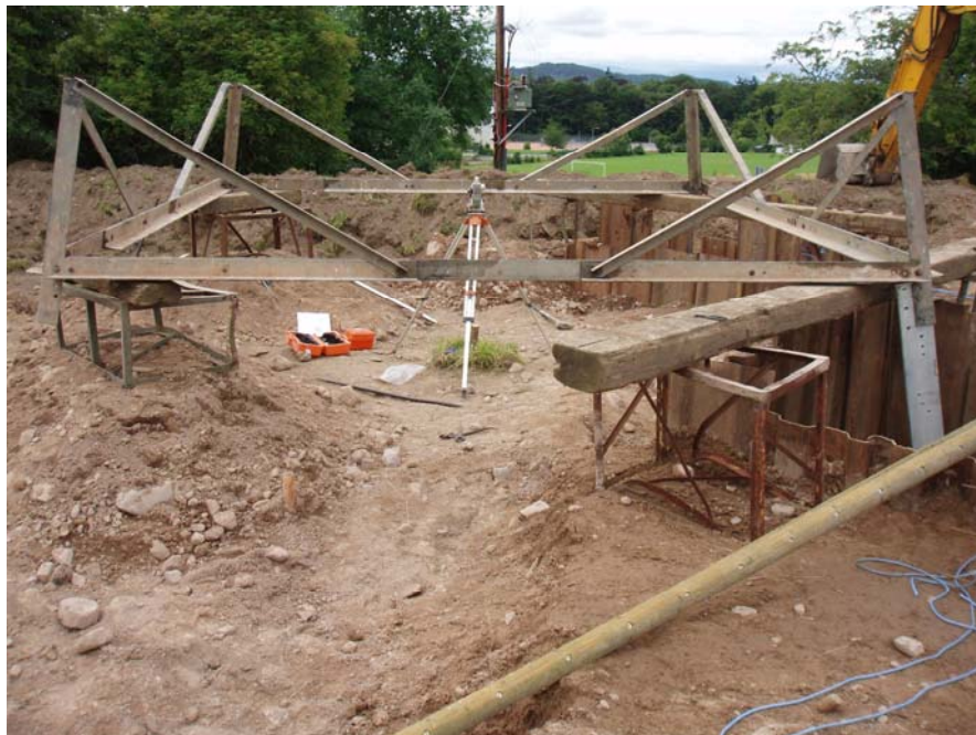
Figure 3.9 – Stub setting template,
