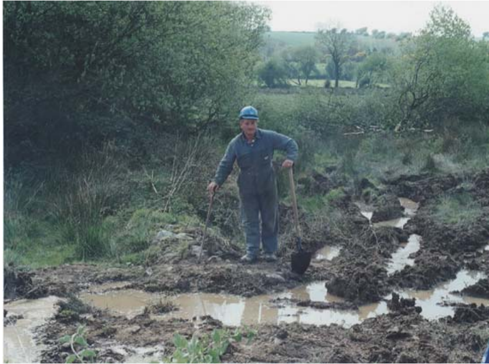
Figure 6.2 – The consequences of failing to provide a temporary access system
