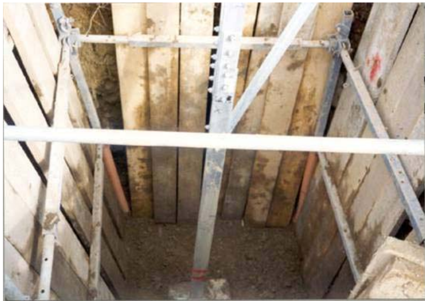
Figure 3.4 – Foundation excavation open sheeting
