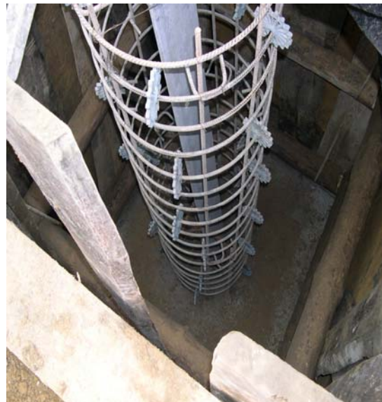
Figure 3.8 - Foundation reinforcement complete with plastic wheel spacers
