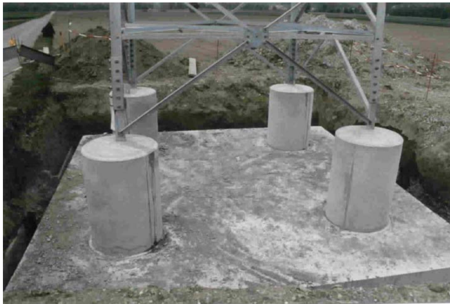
Figure 1.11 – Raft foundations
