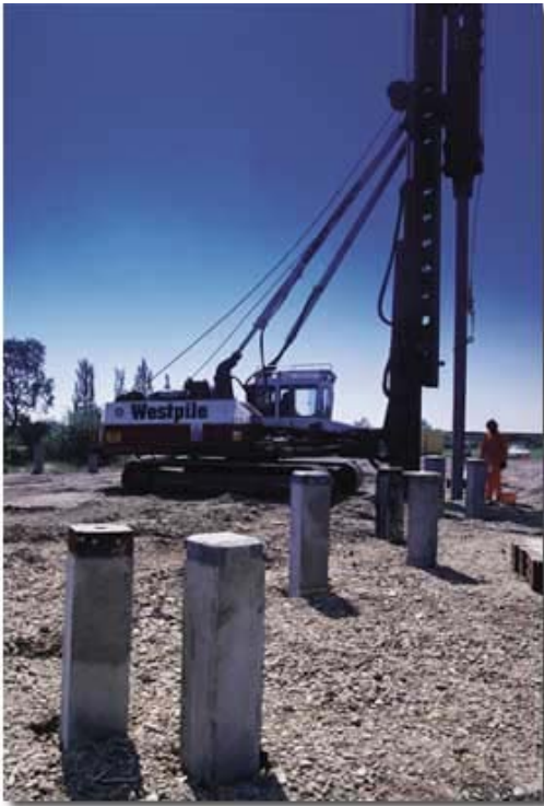
Driven pre-cast concrete piles
