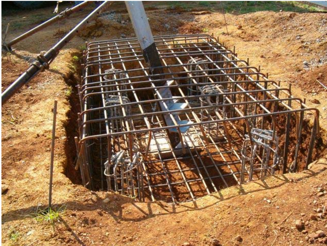
Figure 3A.7c – Auger-pile foundations before concreting of the pile cap
