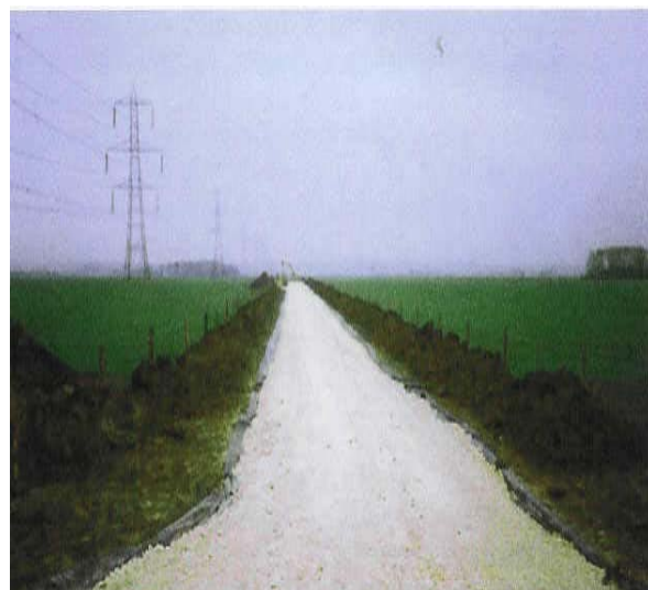
Temporary stone roads
