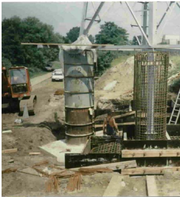
Figure 3A.11c – Bored pile 2 x 1.2 m diameter per leg, details of pile cap and chimney extension 110 kV lattice steel towers ~ Germany
