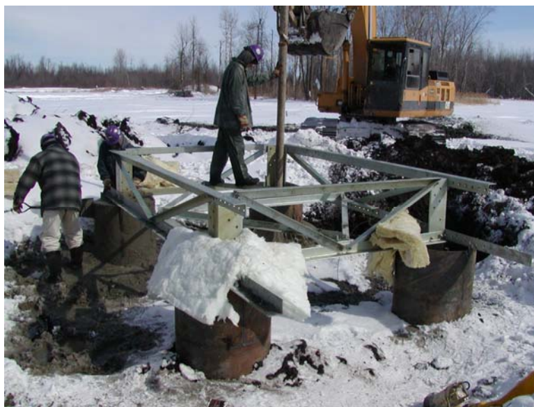
Figure 3.15 – Cold weather concreting, note use of thermal insulation
