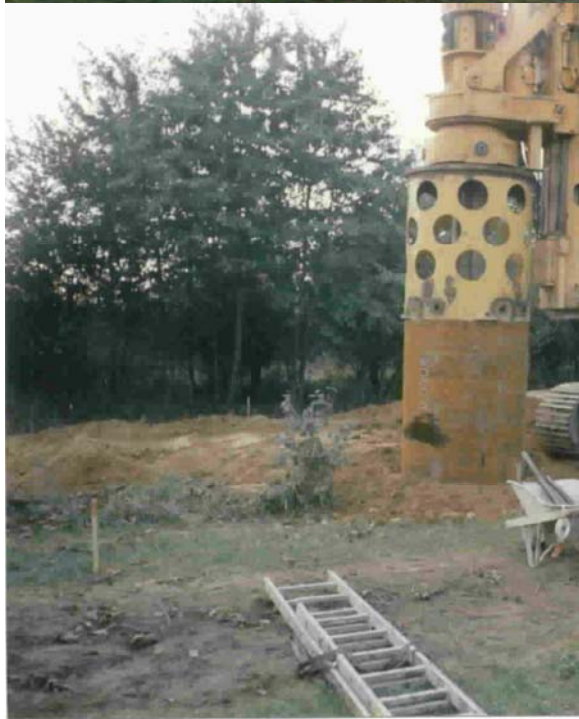
Figure 3A.10 – Details of bored pile installation equipment ~ 1.3 m diameter piles Germany
