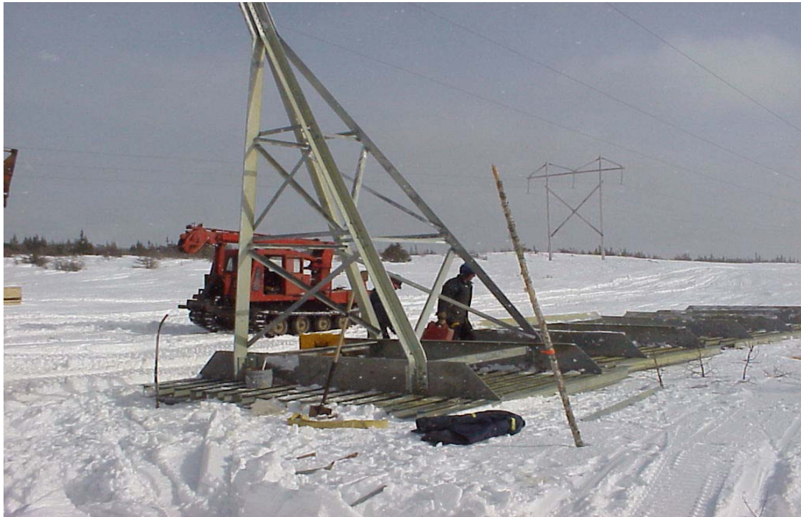
Figure 3A.9a – Assembly of steel grillage foundations for 230 kV OHL - Newfoundland
