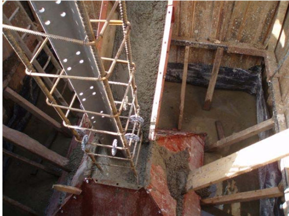
Figure 3.11 – Steel formwork Concreting using chutes
