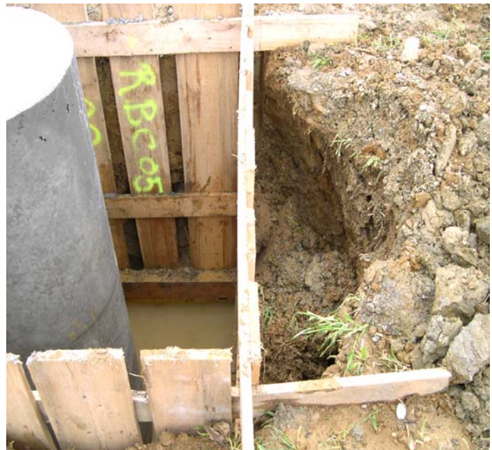
Figure 5.5 – Failure of surrounding soil
