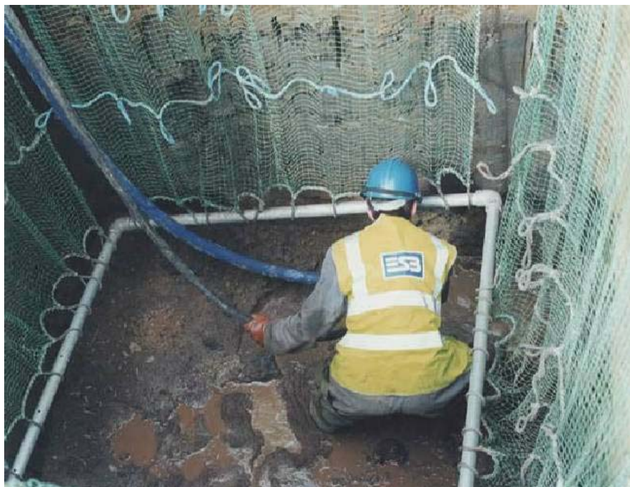
Figure 3.6 – Foundation excavation side support using netting frame
