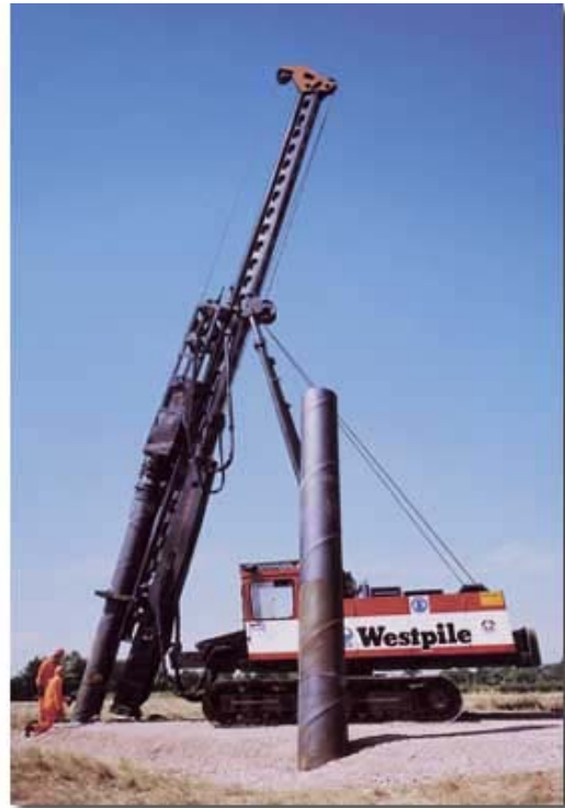
Driven steel tube piles
