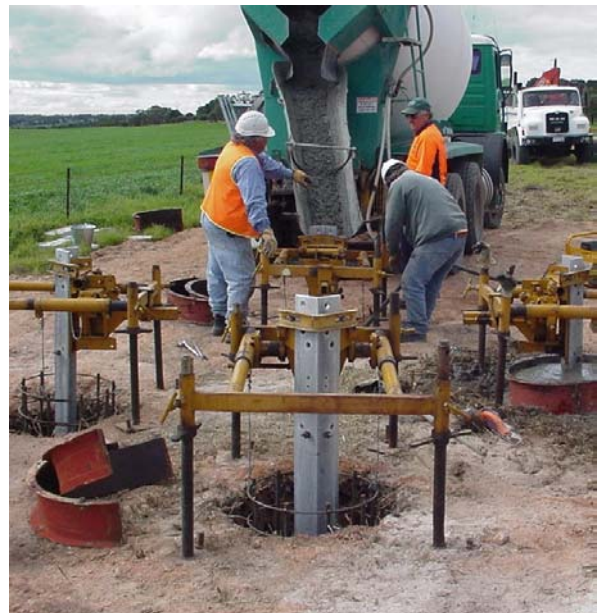
Figure 3.12 – Disposable formwork
