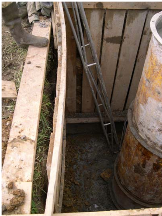
Figure 5.4 – Inadequate support of sides of excavation
