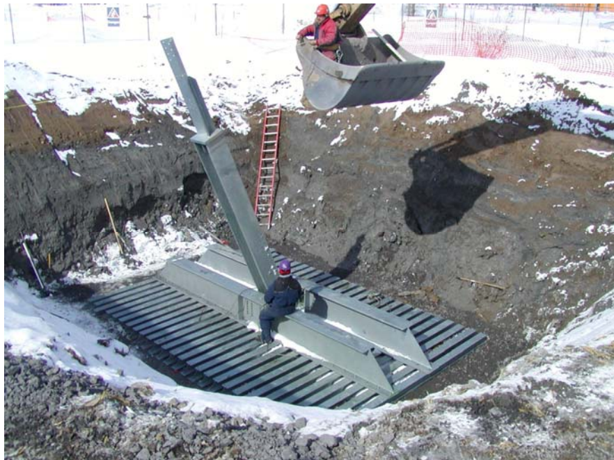
Figure 1.6 – Typical grillage foundations
