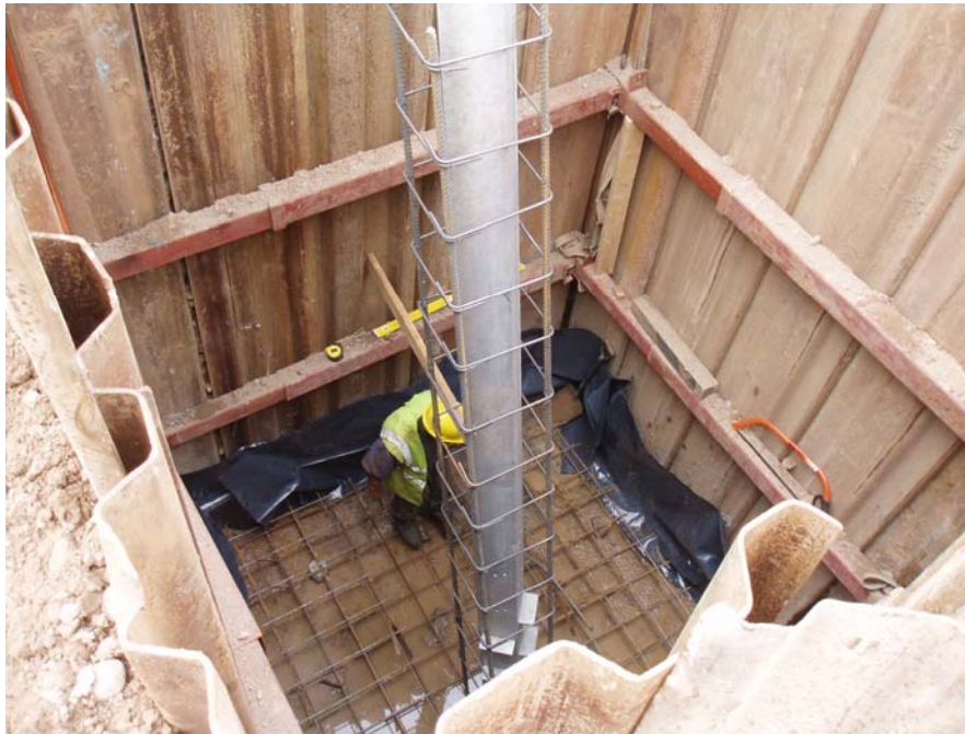
Figure 3.5 – Foundation excavation close sheeting using steel trench sheeting
