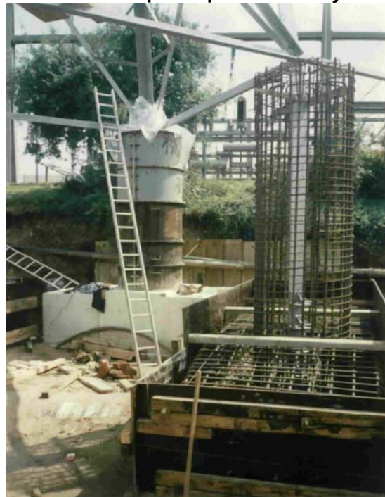
Figure 3A.11c – Bored pile 2 x 1.2 m diameter per leg, details of pile cap and chimney extension 110 kV lattice steel towers ~ Germany
