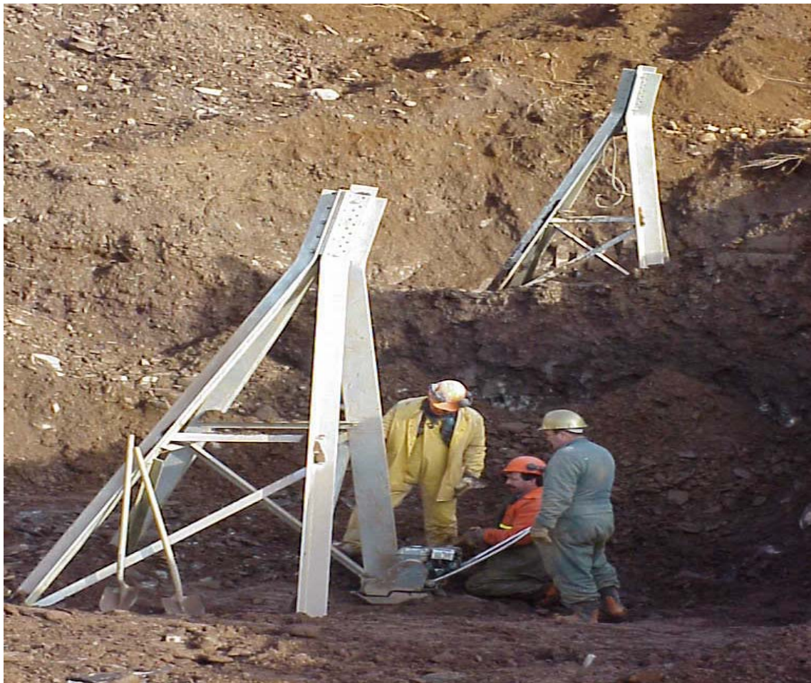
Figure 3A.9b – Compaction of the backfill around the steel grillage foundations
