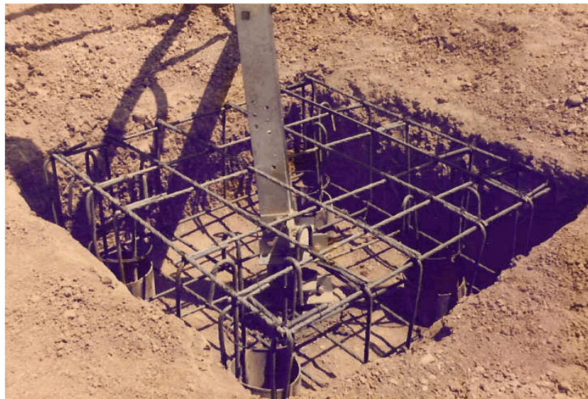
Figure 3A.8 - Foundation Installation - Driven steel tube piles - pile cap
