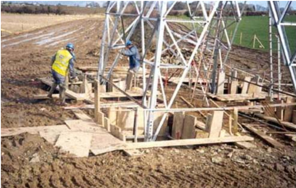
Figure 3.10 – Stub setting using the bottom panel of the tower
