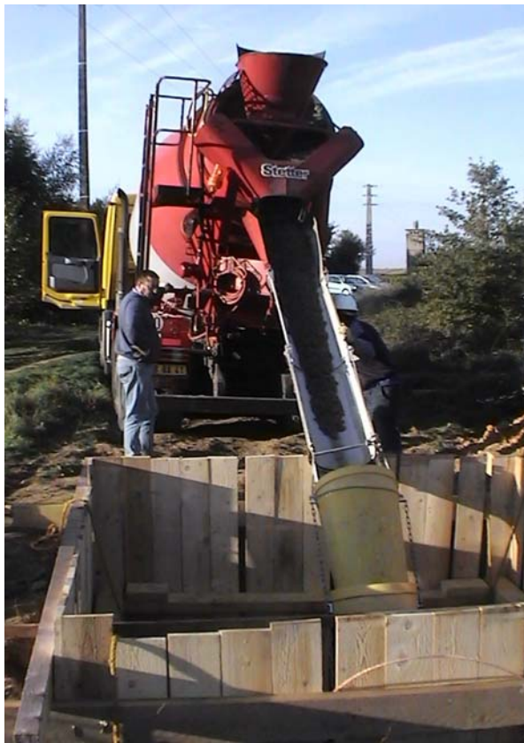
Figure 3.13 – Concreting using chutes
