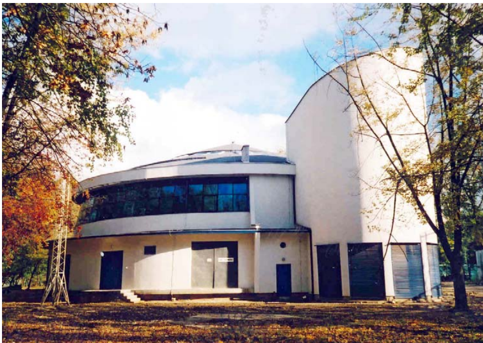
Figure A2-3: Warszawa-Batory Substation after Modernization.
