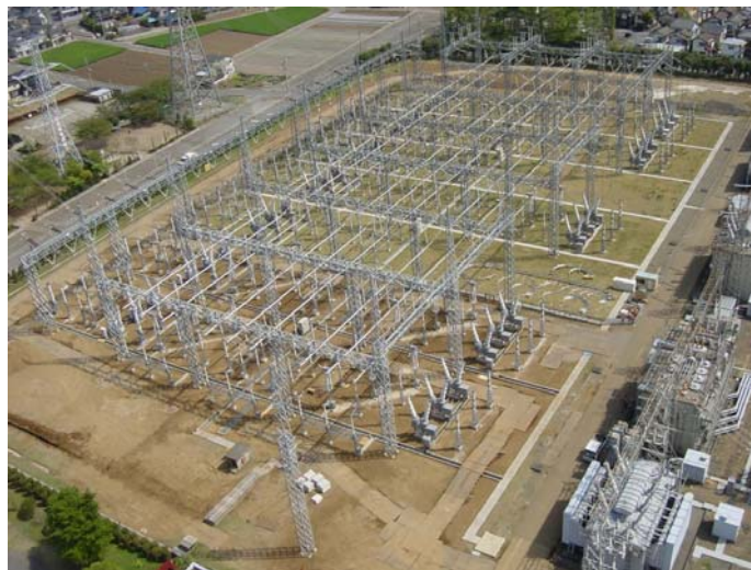
Figure A6-2: The Completed Rehabilitation Project with Suspended Aluminum Tube Bus System
