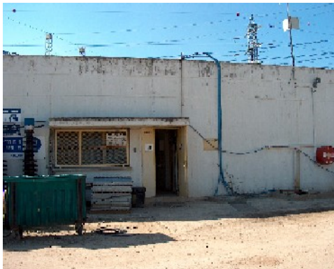
Figure A4-4: Old Control Building
