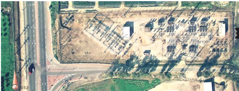
Figure A4-1: Substation General View
