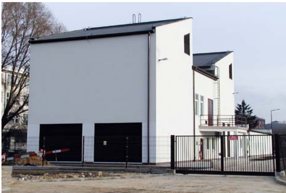
Figure A2-6: Warszawa-Zachodnia Substation after Modernization.
