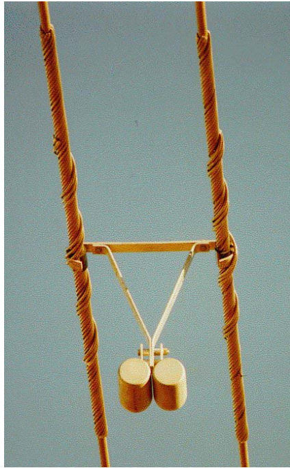
Figure 8.35: Detuning pendulum installed on a twin bundle conductor in Nebraska [Pon and Havard, 1994]
