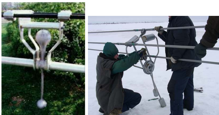
Figure 8.42: Photograph of the torsional damper and detuner (TDD) installed on a twin (left) or triple (right) bundle line [Lilien and Vinogradov, 2002]
