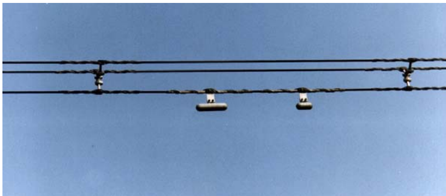
Figure 8.36: Detuning pendulum installed on a triple bundle conductor in Slovakia [Pon and Havard, 1994]
