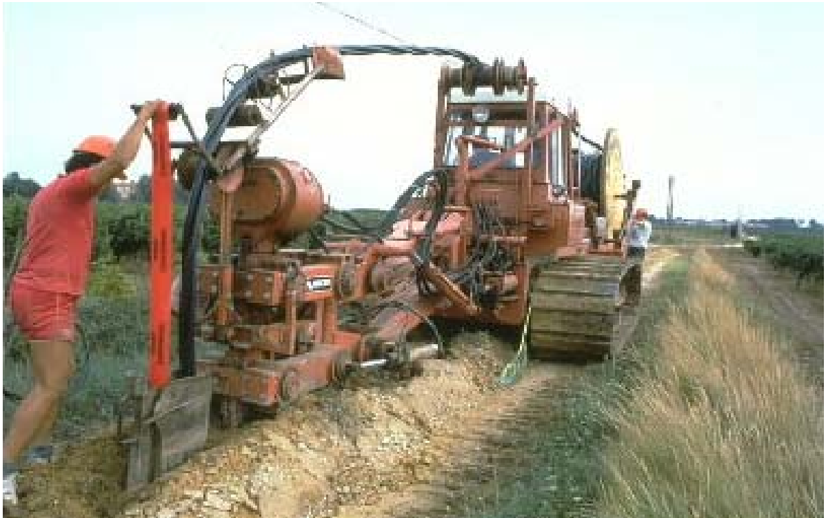
Figure 3.19: Mechanised laying of a 20 kV cable bundle
