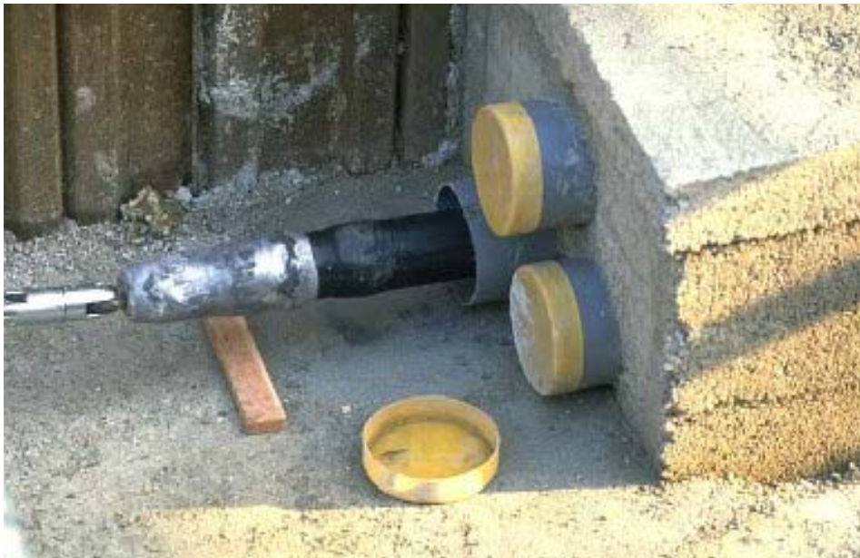
Figure 3.10: Cable being pulled through a pre-installed plastic duct
