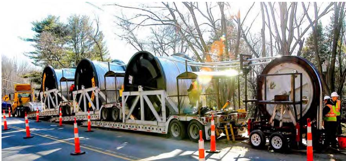
HPFF Cable Installation
