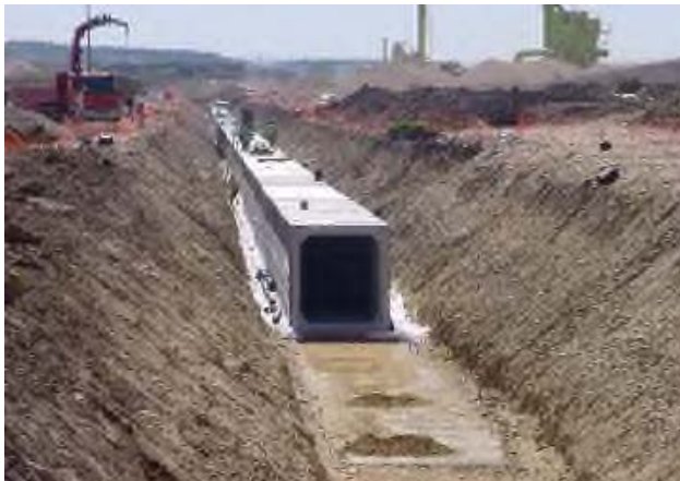
Tunnel under construction
