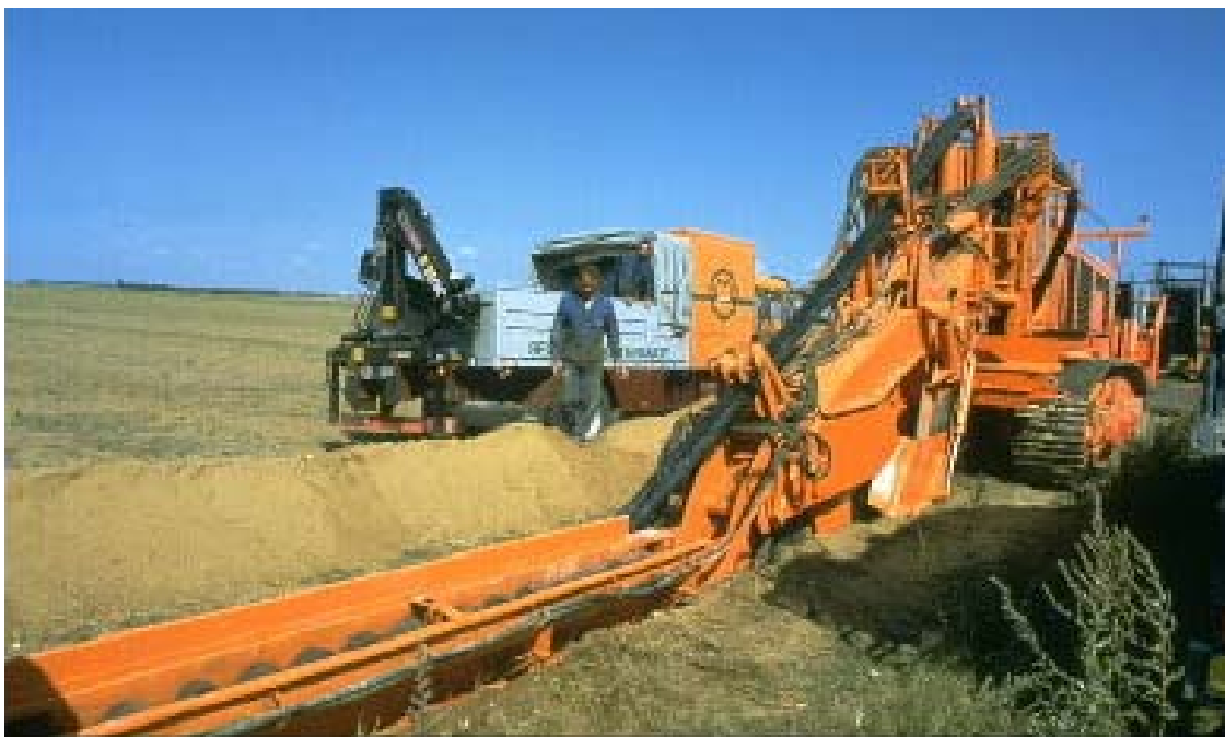
Figure 3.20: Mechanised laying of 63 kV cable ducts
