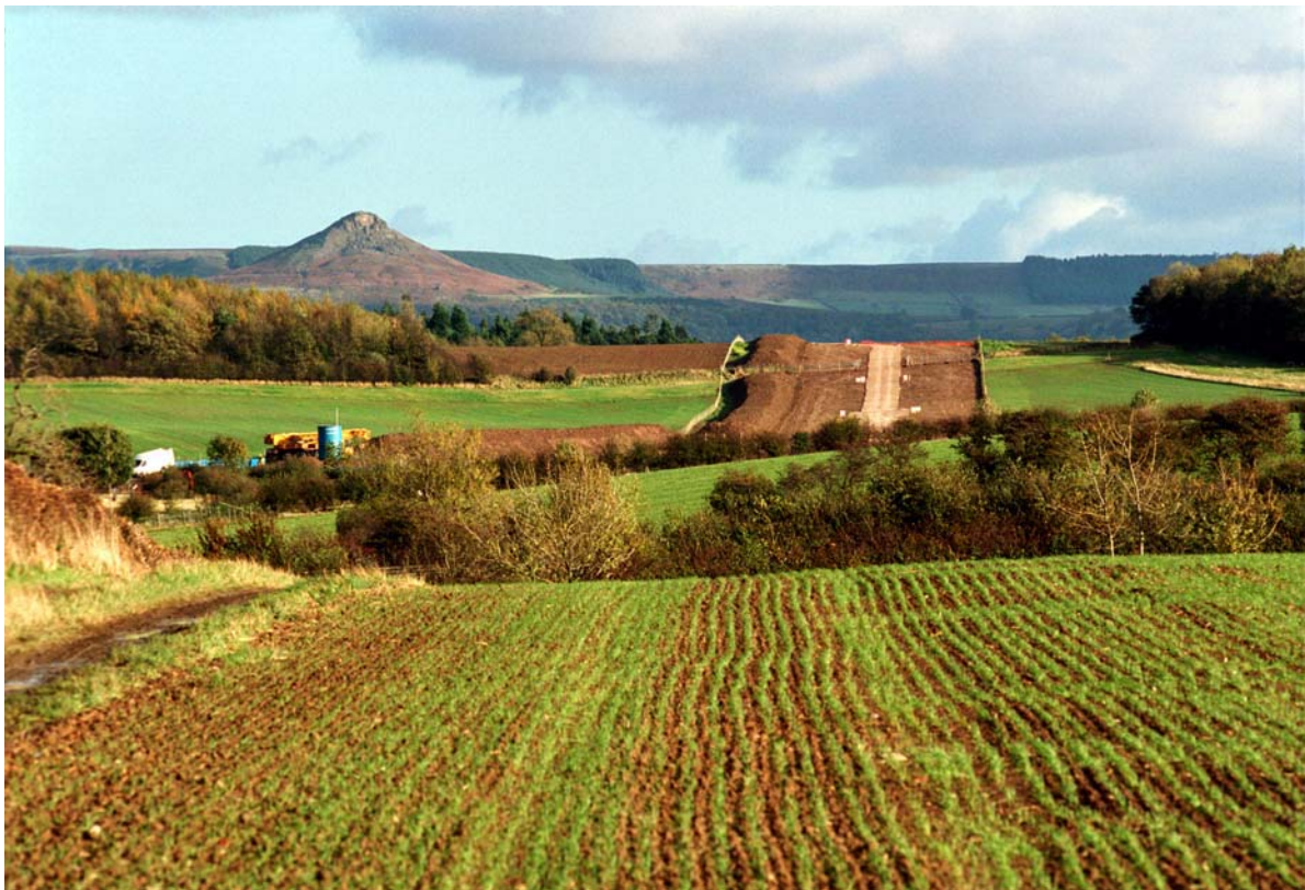
Figure 3.15 Construction swath for the Nunthorpe-Newby 400 kV cables in the UK. Further details on this installation are given in Appendix G.
