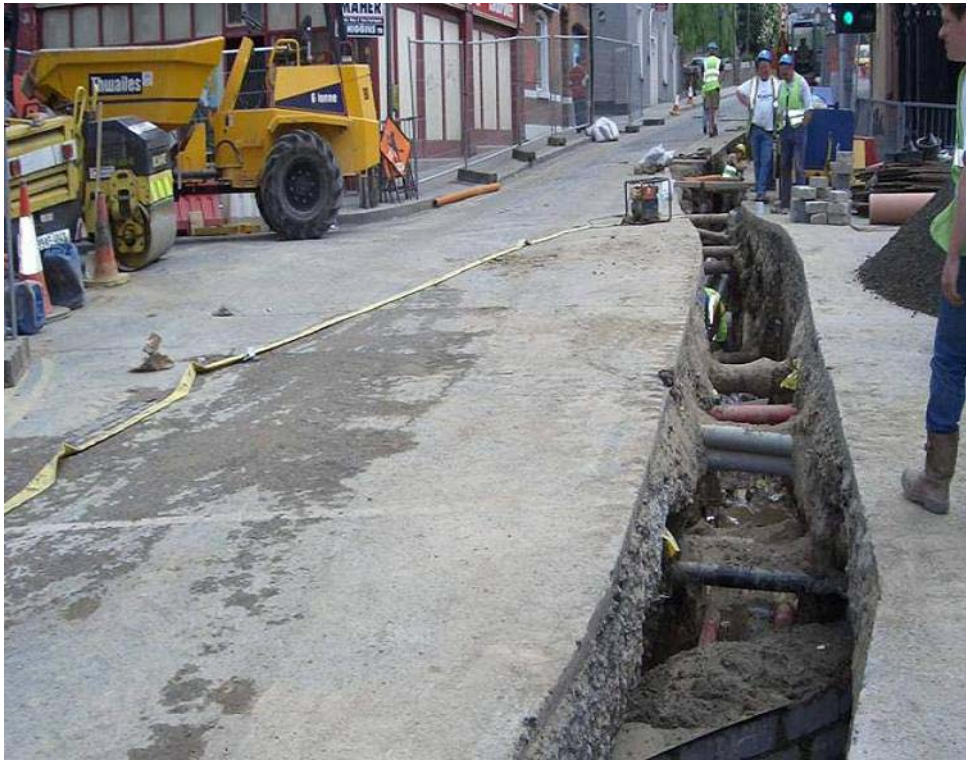
Figure 3.8: 110 kV cable trench in an urban street
