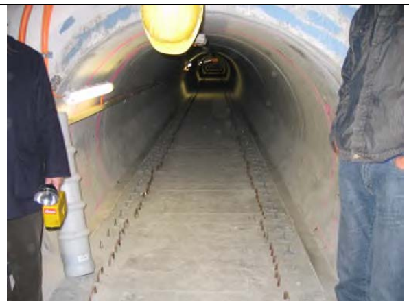
Fig. 5: Picture after completion, covering of bolted concrete blocks
