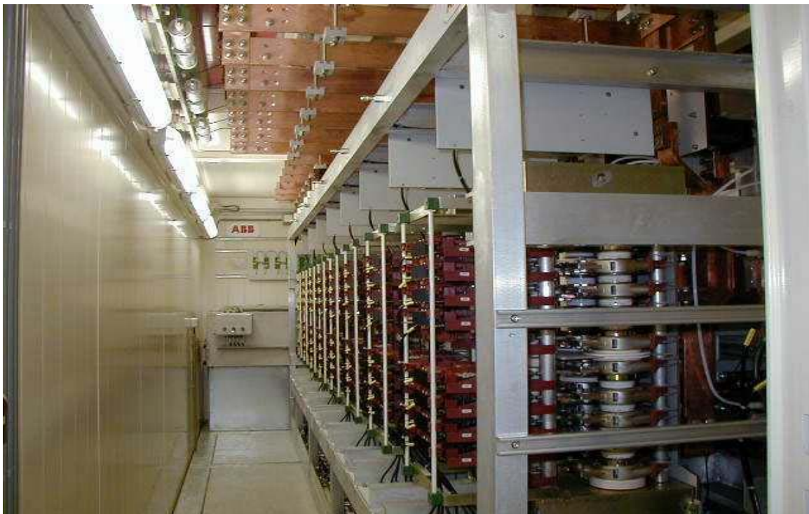
Figure 5-8: Back-to-back intertie based on the NPC IGCT PEBB [87]
