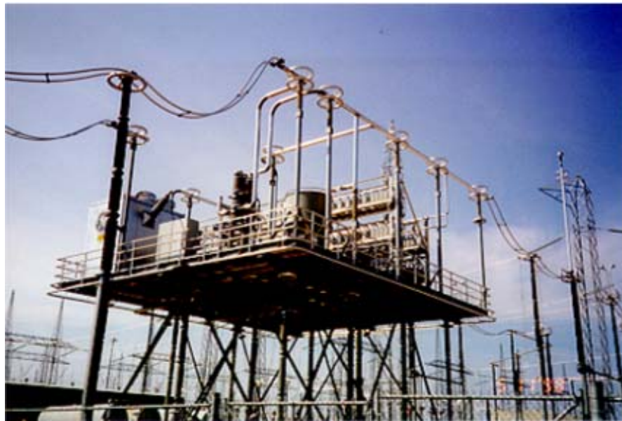
Fig 9.1-1 Example of a 735 kV SC Bank
