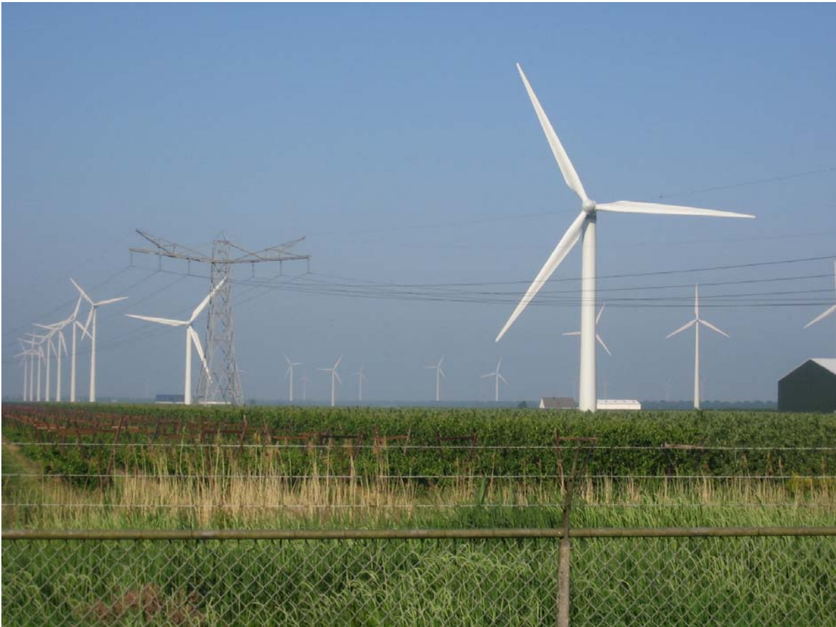
Fig. 21 Windmills in the Netherlands connected to a separate 20 kV-network
