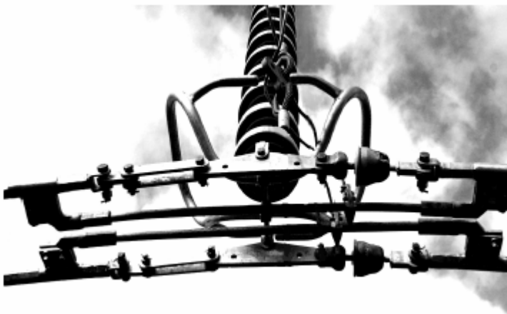
FIGURE XVII. SEMI TENSION SET ARRANGEMENT [10]
