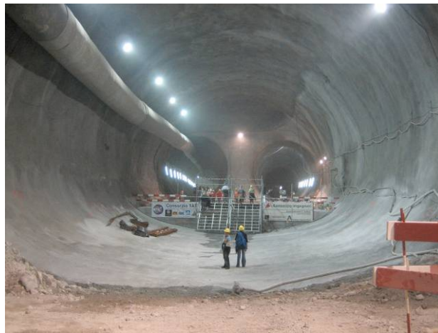
Figure 26: Gotthard Tunnel, Switzerland, double rail track tunnel
