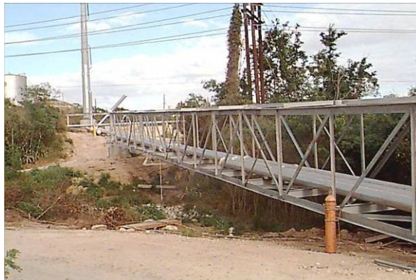
Figure 16: 362 kV GIL , nominal voltage of 230 kV and continuous current of 3000 Amps
