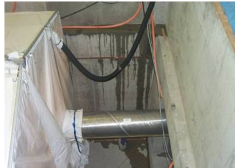
Figure 62: Bringing in the GIL Section into the Welding Area
