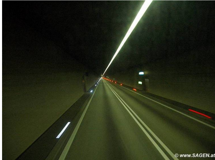
Figure 25: Arlberg Road Tunnel between Tirol and Vorarlberg, Austria
