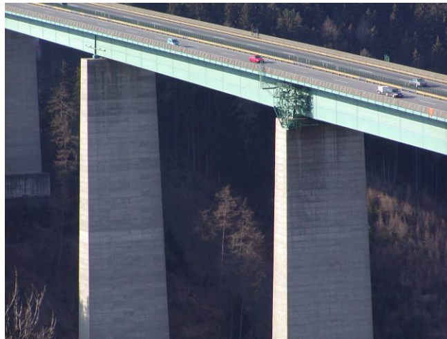
Figure 31: Europe Bridge, Austria 185 m height, detail
