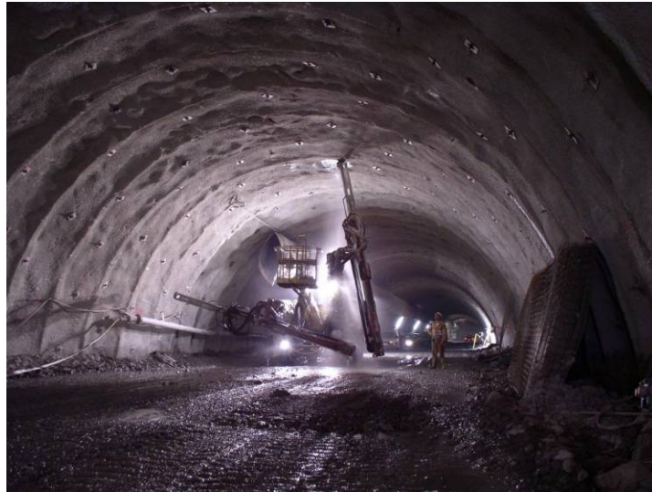
Figure 22: Innsbruck Nordumfahrung Tunnel, Austria, double track rail tunnel
