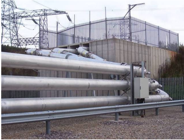
Figure 14: Transfer point above ground to trench installation
