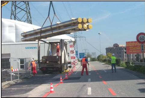
Figure 59: Delivery of Transport Units at Preassembly Area
