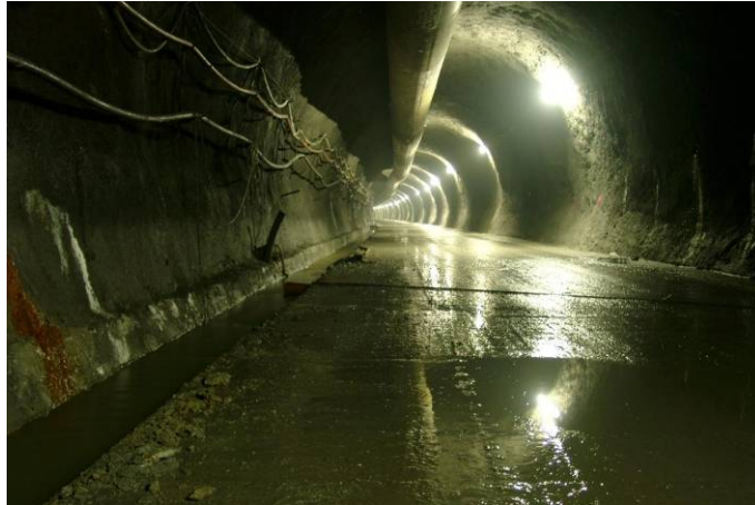
Figure 29: Service or pilot tunnel
