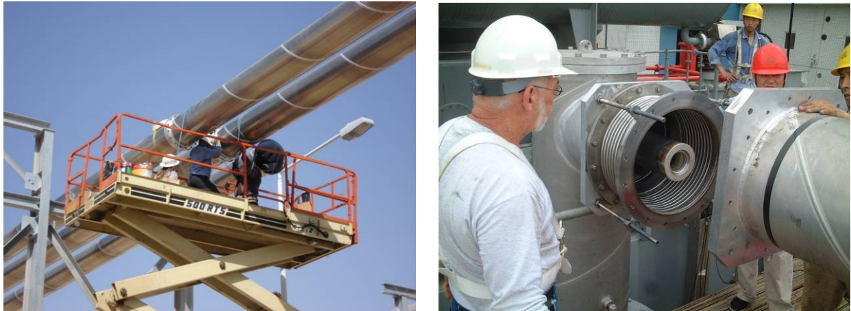
Figure 46: Installation of section of busbar on site
