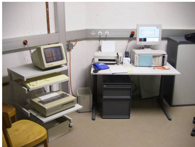
Figure 58: Monitoring room for the data connection to the operation centre
