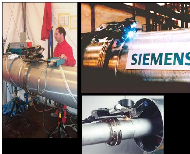
Figure 63: Orbital welding machine for enclosures and phases
