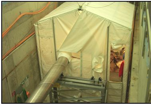
Figure 61: Welding Area in the Tunnel
