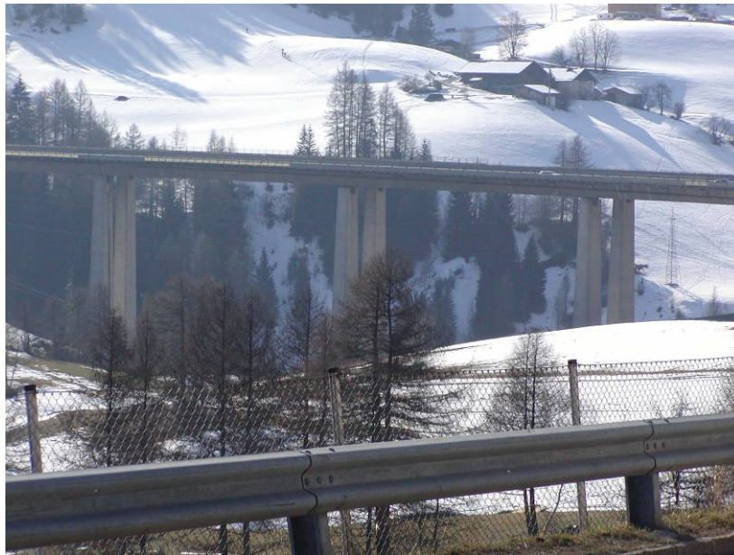
Figure 32: Gschnitztal Bridge, Austria approx. 80 m height, bended
