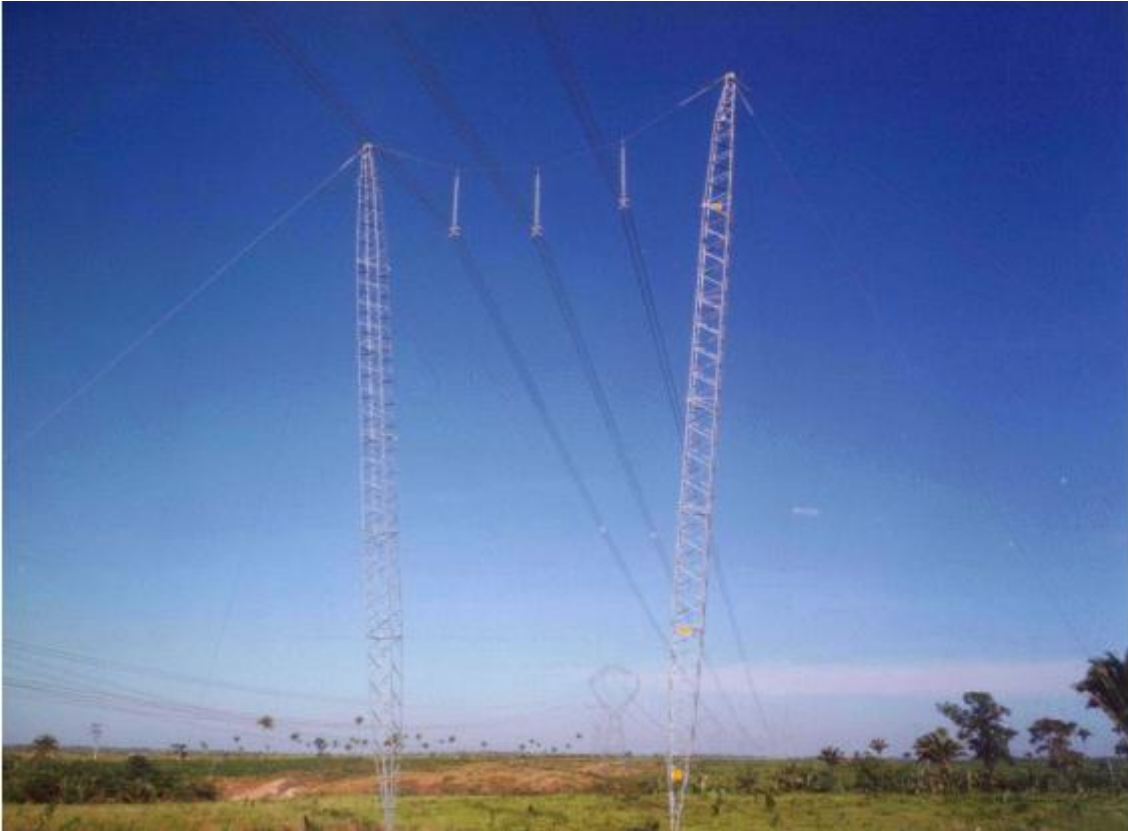
Figure 1.3 - 500 kV Compact cross rope suspension tower
