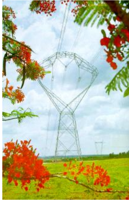
Figure 1.1 - 500 kV compact racket tower in Brazil
