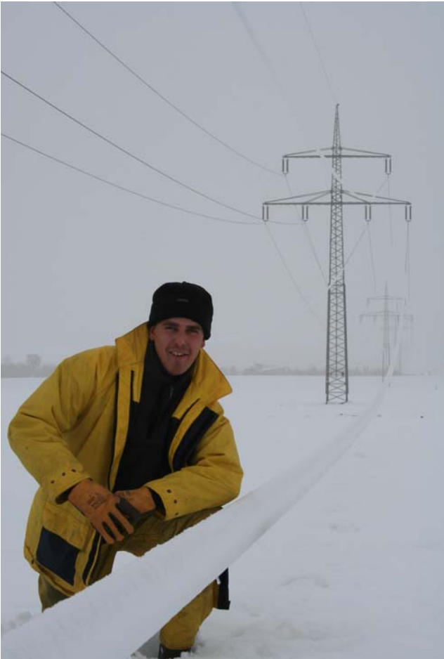
Figure 6 – Snow accretion after the wet snow storm on November 24-25, 2005, Germany (E.ON)
