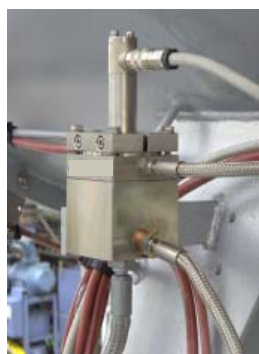
Figure 5 Buchholz gas volume sensor
