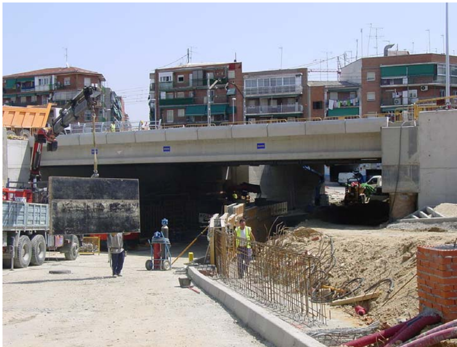
Picture 2. Widening of a tunnel below the line.
