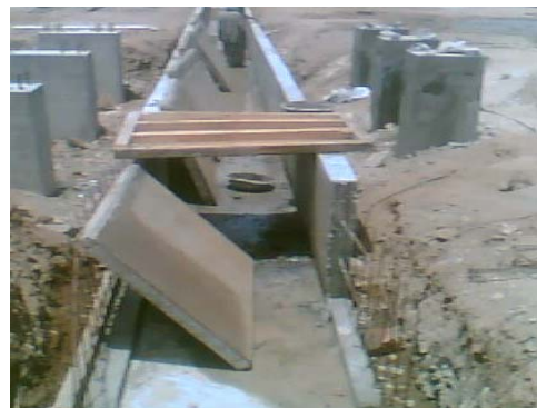
Figure: 2-4 RCC trenches
