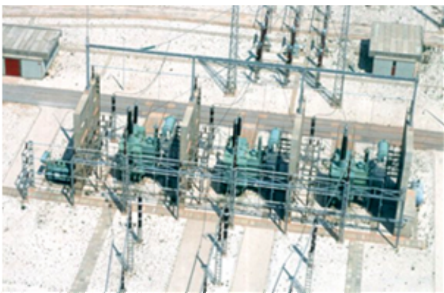
Figure B-8-3: Conventional three-phase bank solution
