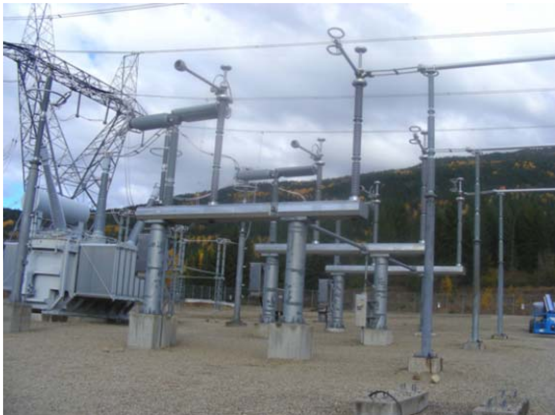
Figure B-7-2: After conversion
