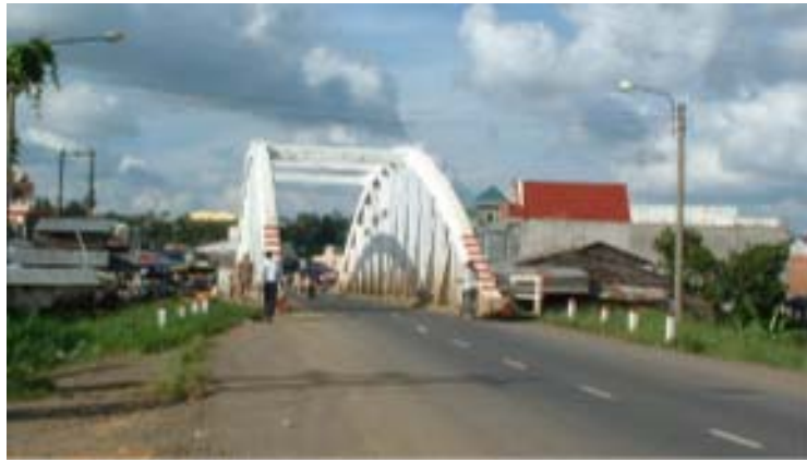
Figure 4-3 Pre-road survey of bridge for transformer transportation
