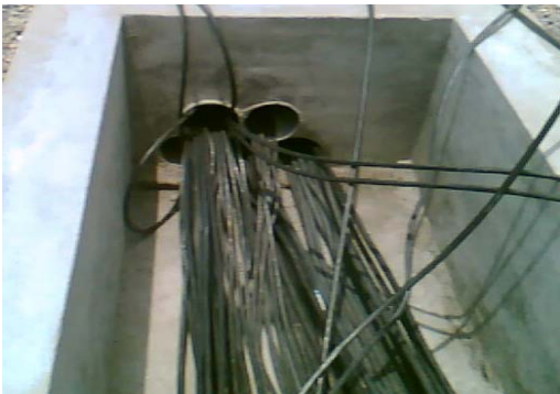
Figure: 2-3 Man Hole for Pipe trenches
