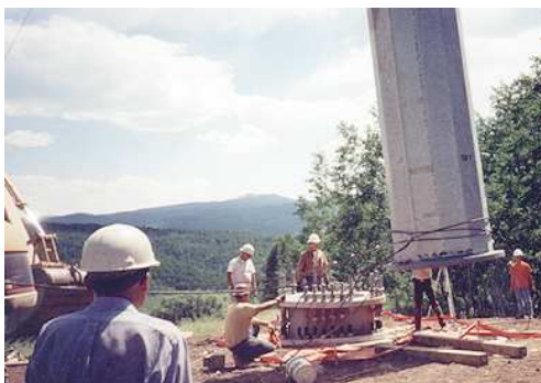
Figure 4: Structure is manoeuvred onto the leveler
