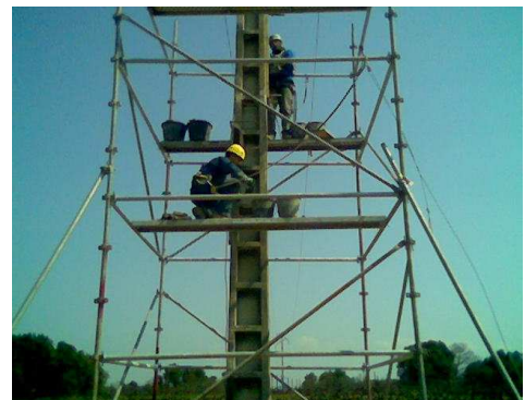
scaffolding installed to facilitate the repair works on a damaged pole
