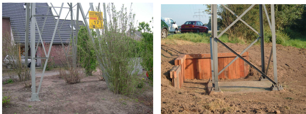
Figure 6-5: Changes of Environment (e.g Raising Soil Around Foundations) will Lead to Refurbishment of Foundations or Soil near Foundations
