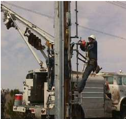
Installation of System to Raise Structure
