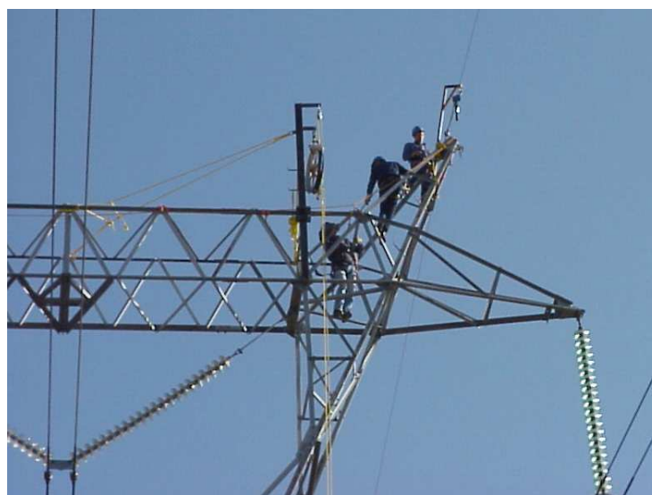
Workers installing optical fibre cable by live line methods
