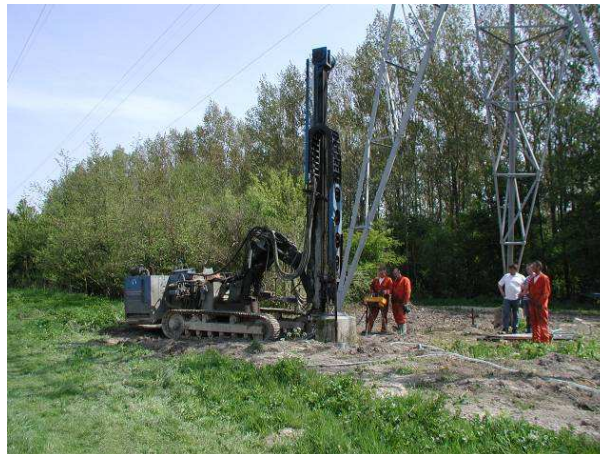
Figure 5-2: Equipment for upgrading foundations
