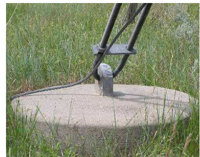
Pier foundation replacement for corroded anchor rods
