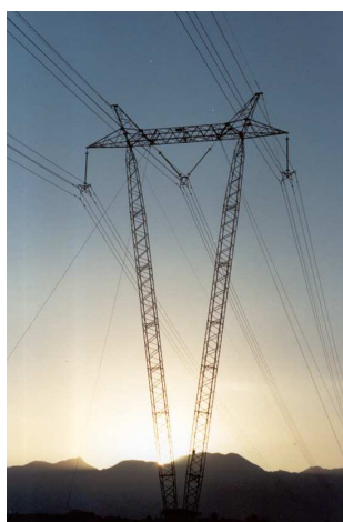
Figure 4-11: 500 kV EXB Transmission Line 744 km Long
