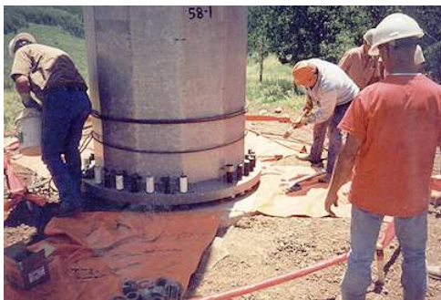
Figure 2: Crew Members remove bolts and place PVC pipe segment over the bolt threads to protect them from damage when structure is lifted off the foundation.
