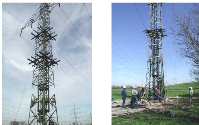
Figure 4-4: Increasing Tower Height
