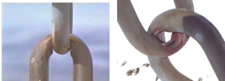
Figure 6-22: Wear at Suspension Bolts
