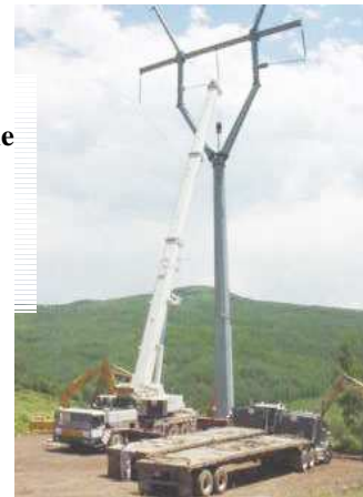
Figure 4: Structure is manoeuvred onto the leveler
