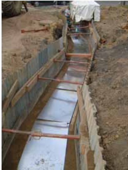
Figure 6.2.27 Sight of the vertical and horizontal plates before refilling the trench.
