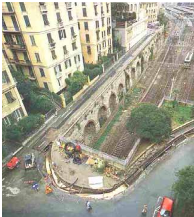
Figure 6.5.3 Aerial view during the pipe installation in Genoa.
