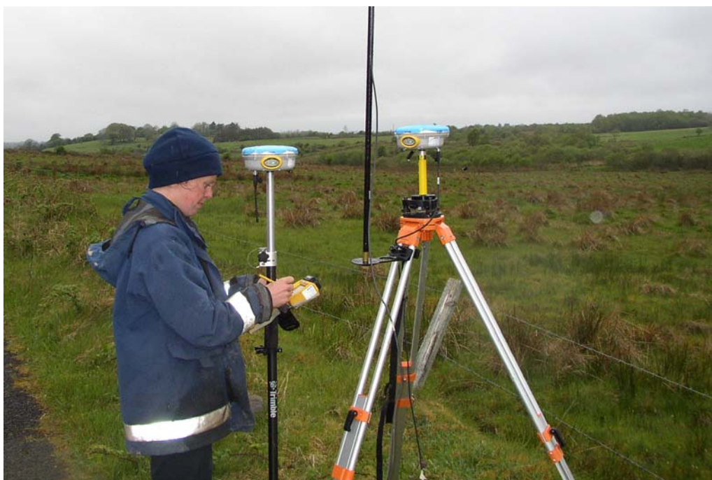
Figure 45 GPS RTK equipment in use for transmission line survey (Source ESB, 2007)
