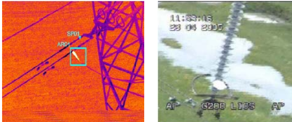
Figure 27. Thermal Infrared (IR) Image left and Ultraviolet (UV) images right recorded from the air. (source Cigre B2/D2-108)
