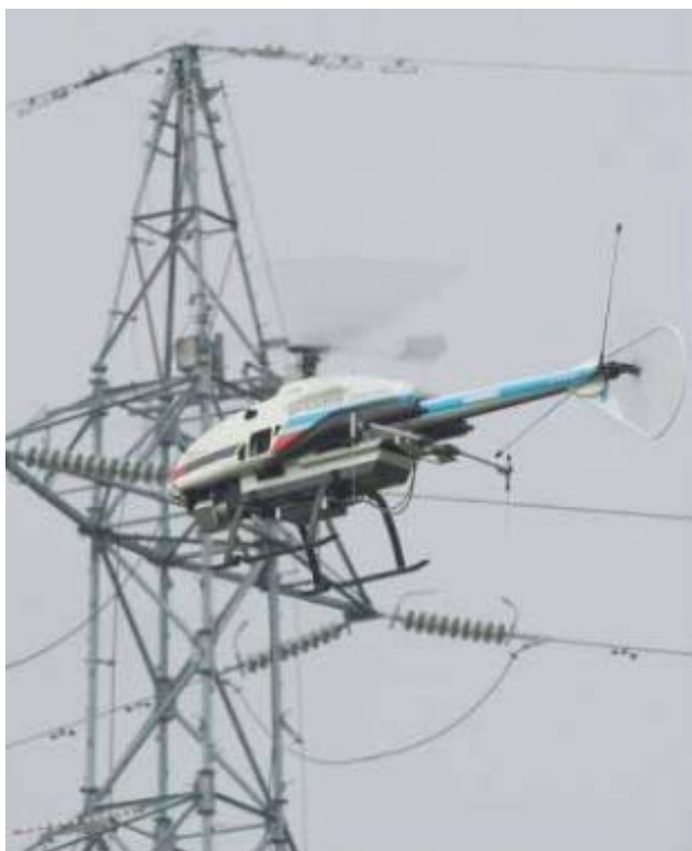
Figure 28. Unmanned inspection using a remote controlled helicopter (source Cigre B2/D2- 106)
