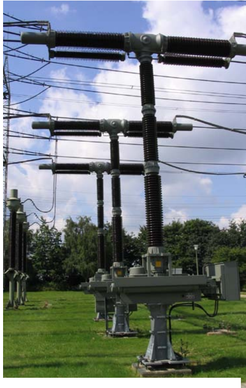
Figure 1 - Two unit circuit-breaker with grading capacitors
