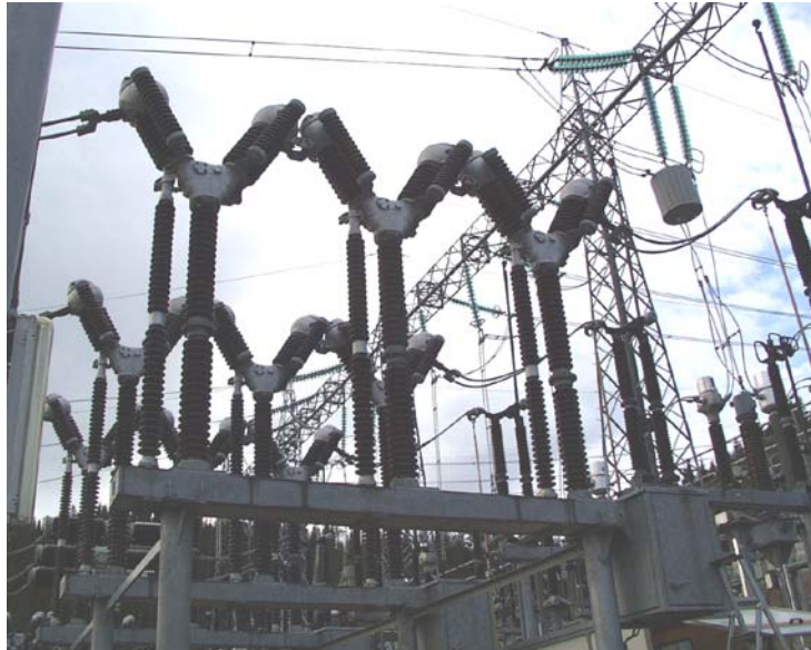
Figure 19 – Circuit-breaker C with six units per pole
