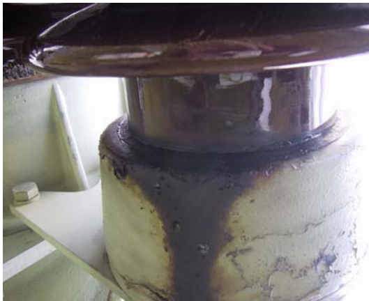
Figure 5 - Typical example of an oil leak from an old AIS grading capacitor (left), and a schematic drawing of a typical flange and sealing arrangement (right)
