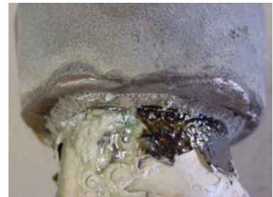
Figure 5.6: Molten end fitting and cement /9/
