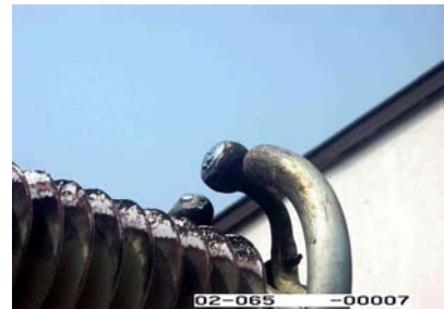
Figure 4.3: Composite post with suitable hardware after 30 kA for 0.5 seconds
