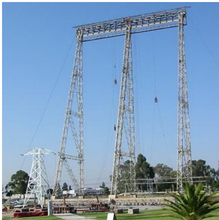
Figure 36: ESKOM Test station facilities.
