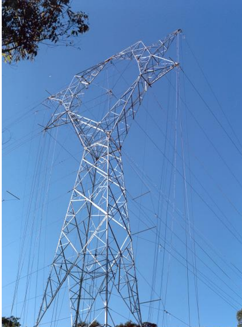
Figure 3 – 500 kV Tower Under Testing
