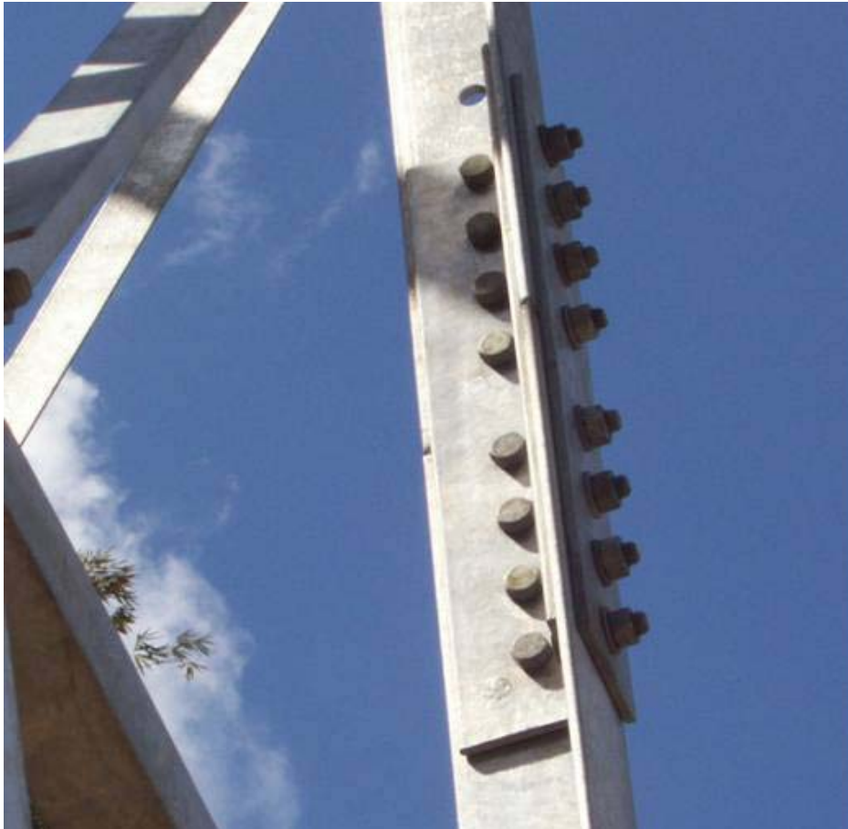
Figure 3.2 – Typical main member’s connections
