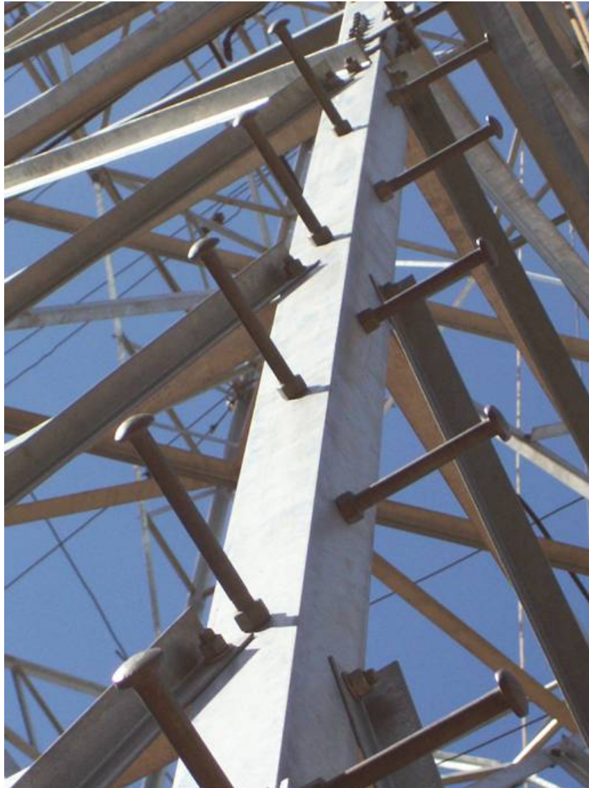
Figure 3.4 – Step bolts assembling
