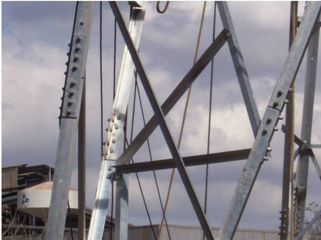
Figure 8.3 – Leg members connections
