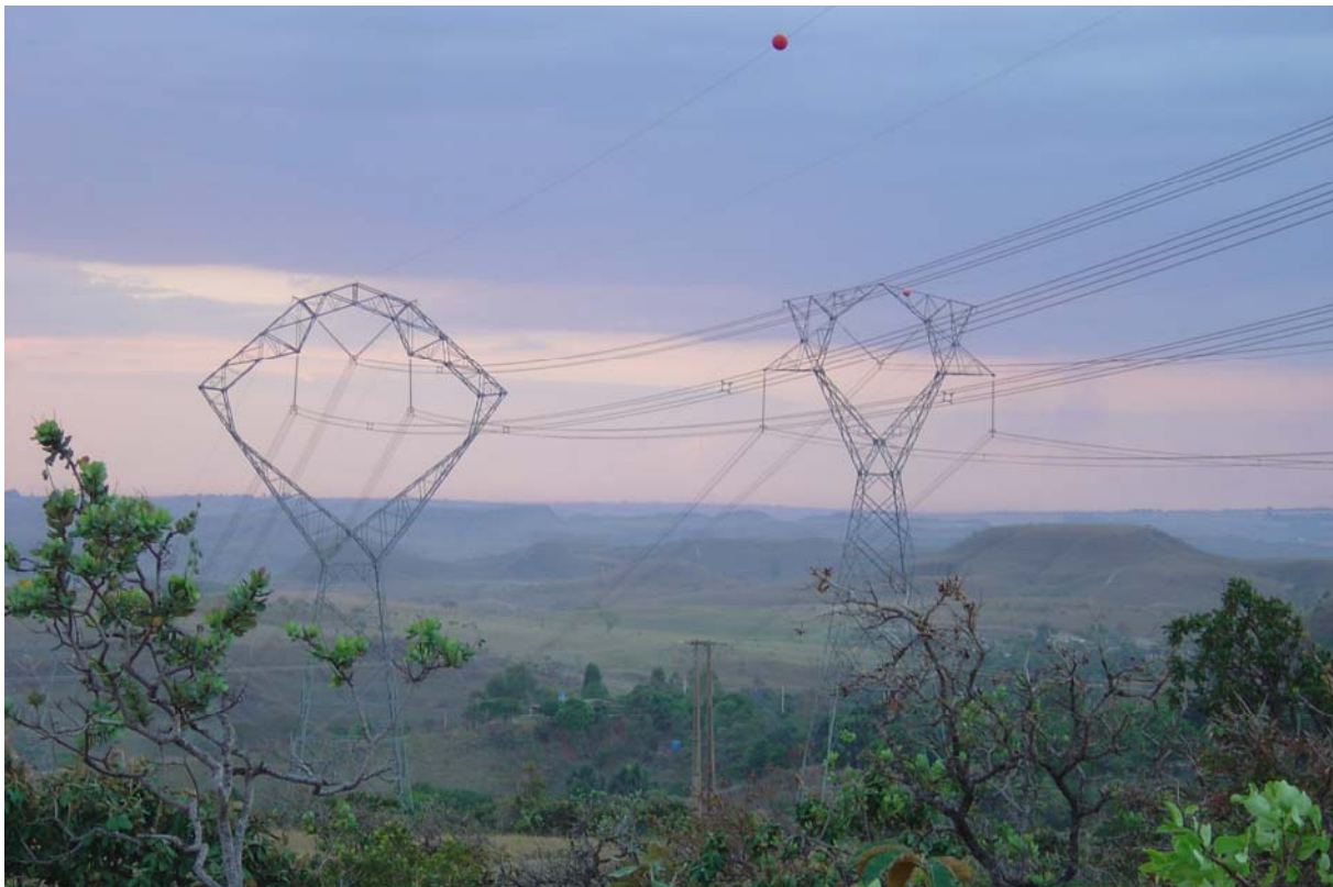
Figure 1 – Different 500 kV Lattice Tower Types
