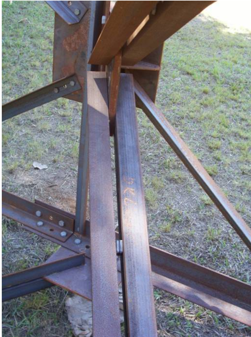
Figure 14.3 – Detailing using double angles
