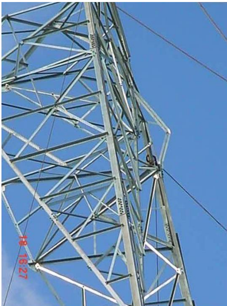
Figure 11.18 – Double angle diagonal buckling
