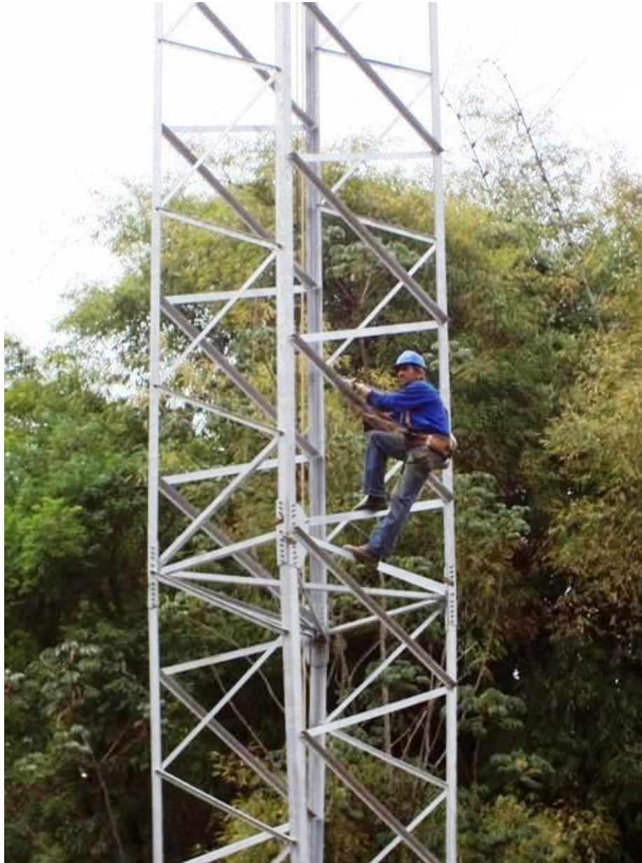
Figure 15.3 – Members reinforced to withstand vertical loads
