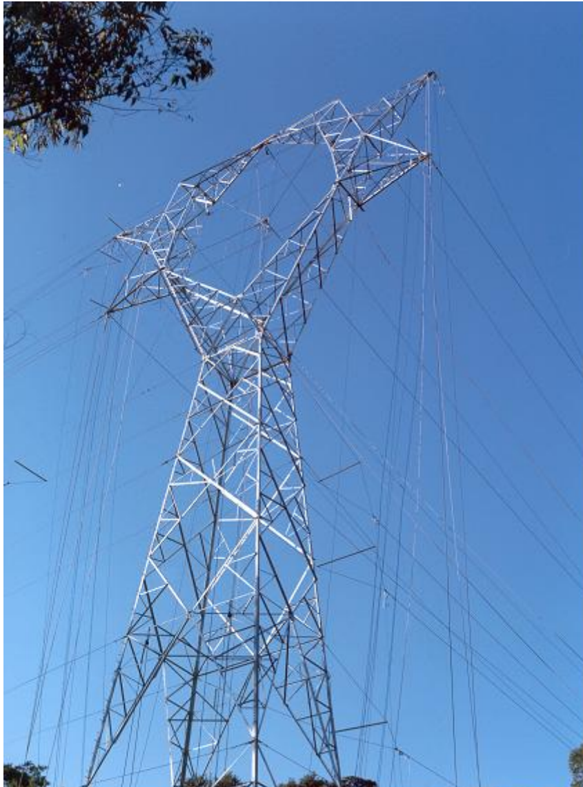
Figure 12.1 – Main and redundant members
