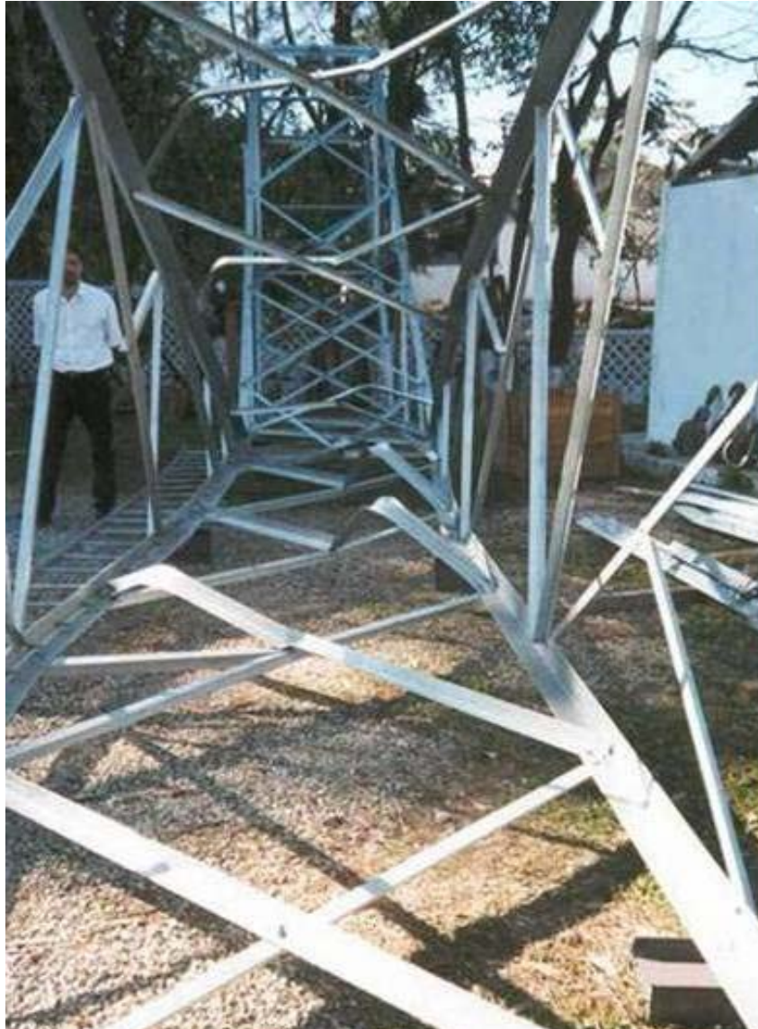
Figure 10.1 – Diagonals buckling during test. See the bracing provided by the tension diagonals.
