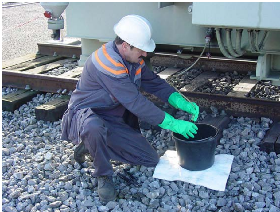
Figure 7: Transformer maintenance– Source: ELIA
