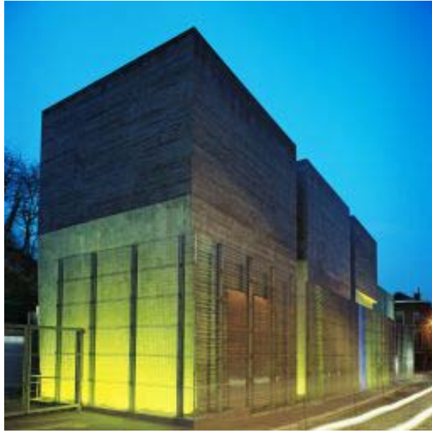
Figure 9: Substation integration– Source: ELIA
