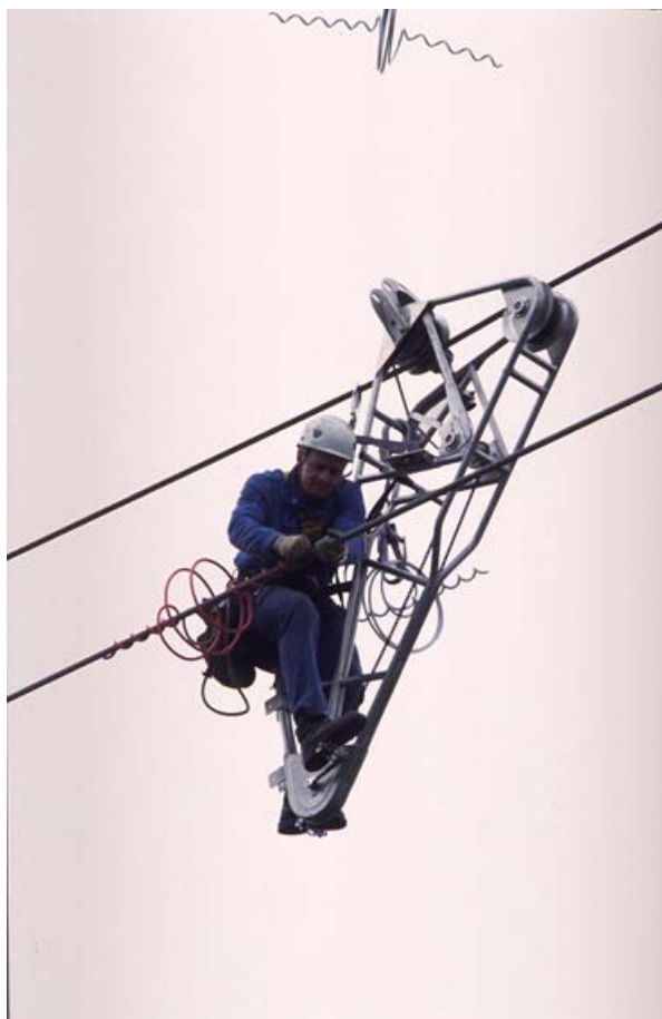
Figure 3: Bird savers spirals implementation on OHL – © Médiathèque RTE / PICART Fabrice
