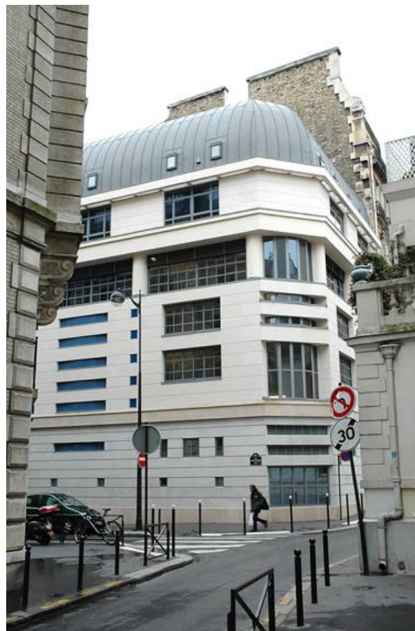
Figure 11: Substation integration in urban area– © Médiathèque RTE / LARVOR Gilles
