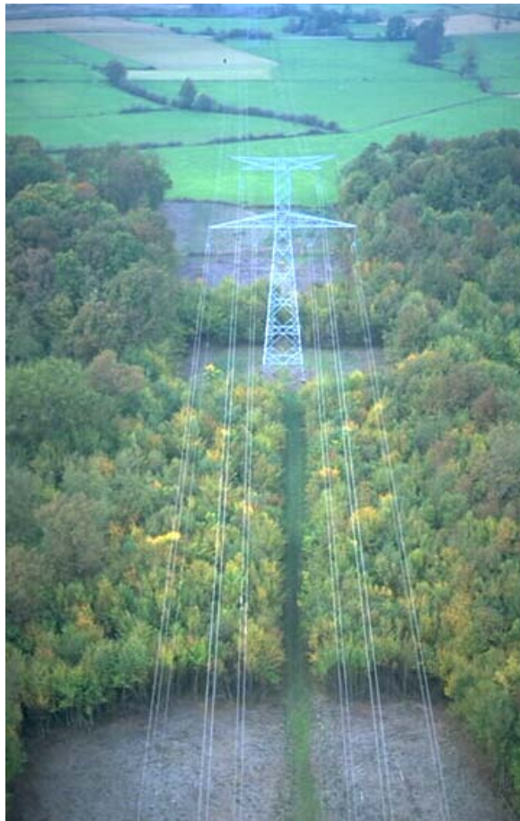
Figure 5: Vegetation management– © Médiathèque RTE
