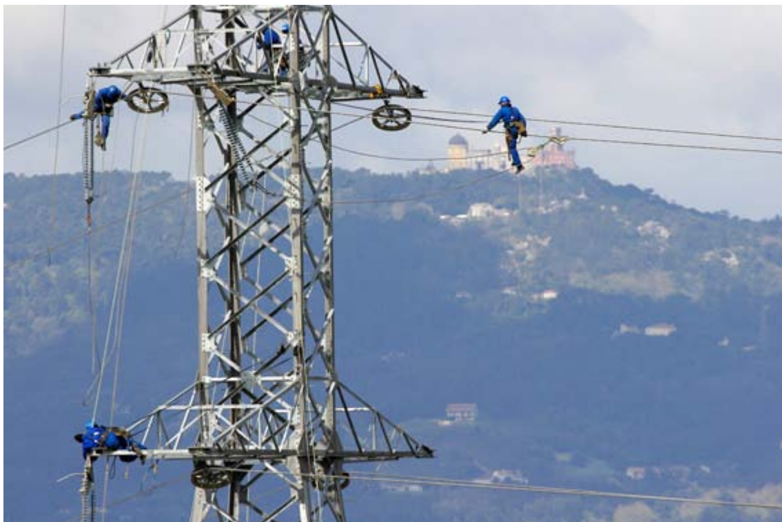
Figure 10: Work on OHL– Source: José Antunes for REN
