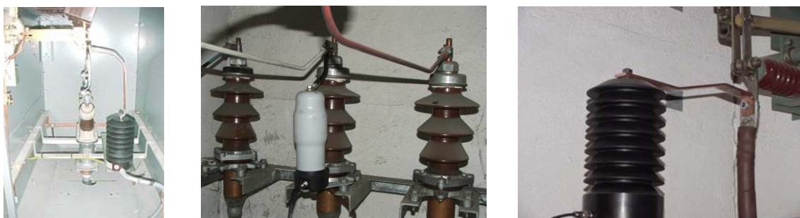
Figure 3-3 Capacitive coupling
