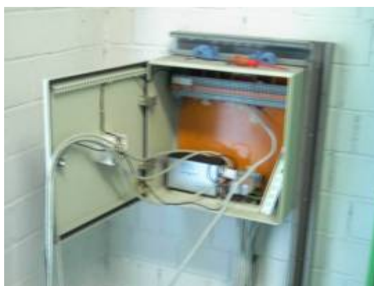
Figure 5-4 : Broadband PLC with RTU-Equipment
