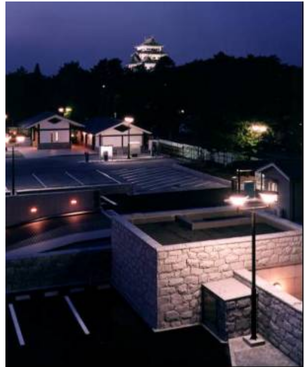
Fig. 4.10.8: Night view of castle tower and buildings of substation
