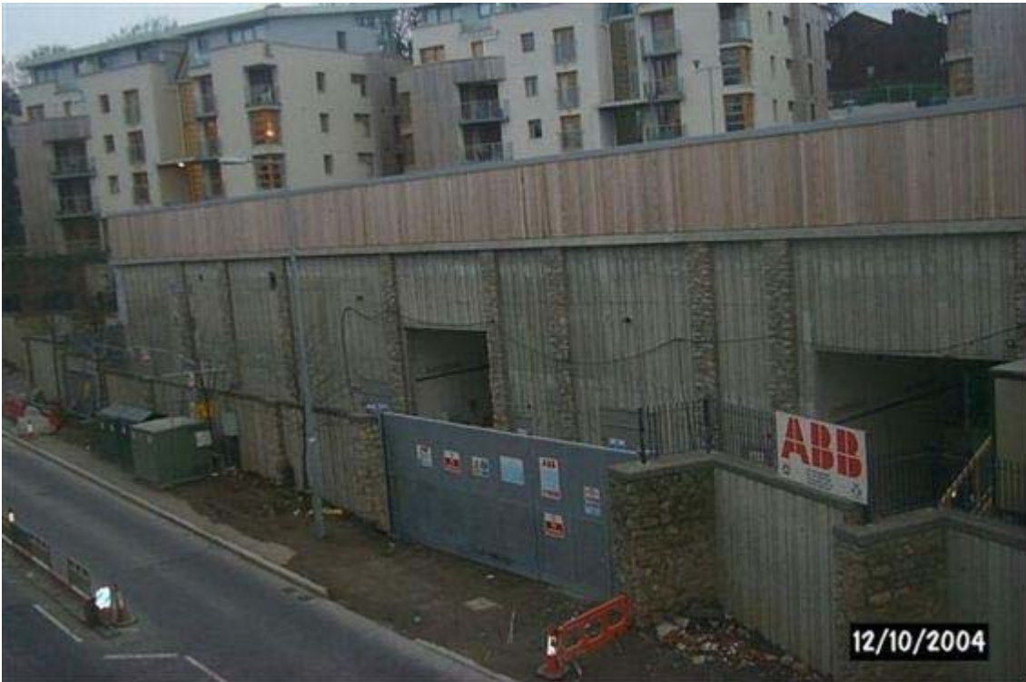
b) During Substation Construction
