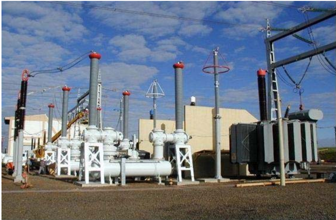
Figure 2.1 Example of Mixed Technology Substation at 550kV
