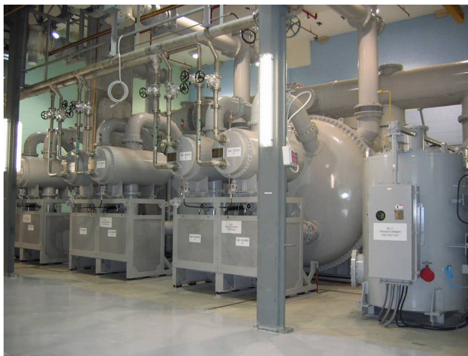
Fig 1. Gas Insulated Transformer, Haymarket, Australia [3].
