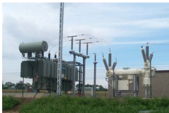
Fig. 2: GIS in/out arrangement
