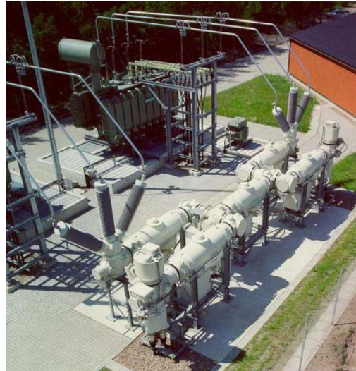
Fig.10: H-scheme with 5 breakers in MTS [9] and outdoor GIS [3]
