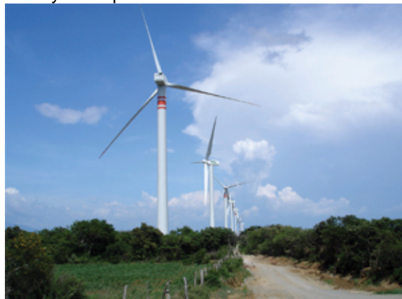
Fig 2. Typical small wind farm array.
