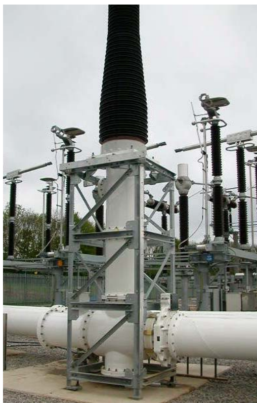
Fig 3. Capacitive voltage transducer [2]
