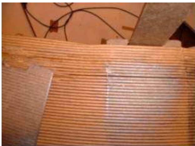
Fig. 1e Copper sulphide deposits found under spacer in failed HVDC transformer, from [18]
