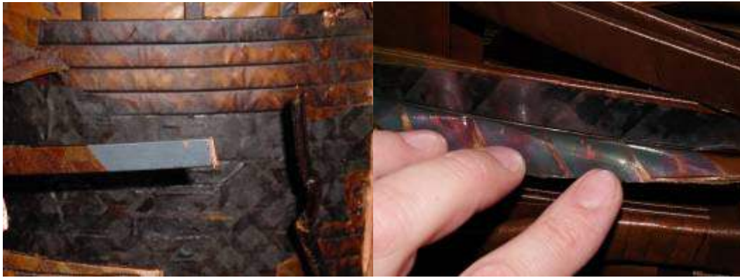
Fig. 1f Conductor and papers from the inspection of a failed unit
