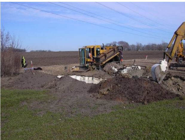
Figure 4.6 Horizontal directional drilling
