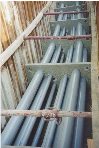
Figure 4.8 Ducts consisting of PE or PVC pipes (left) cast in concrete (right)
