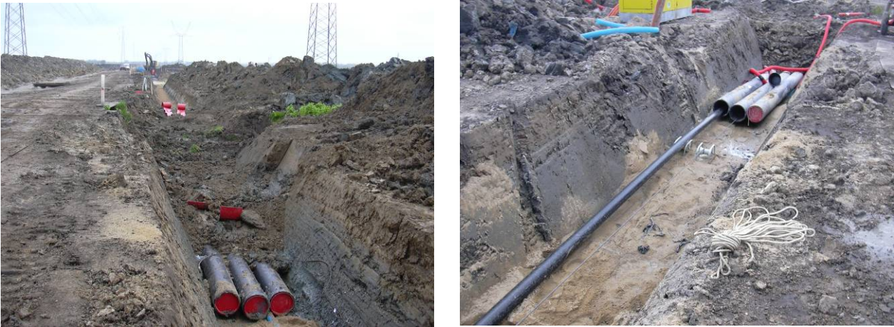
Figure 4.7 Laying in pipes
