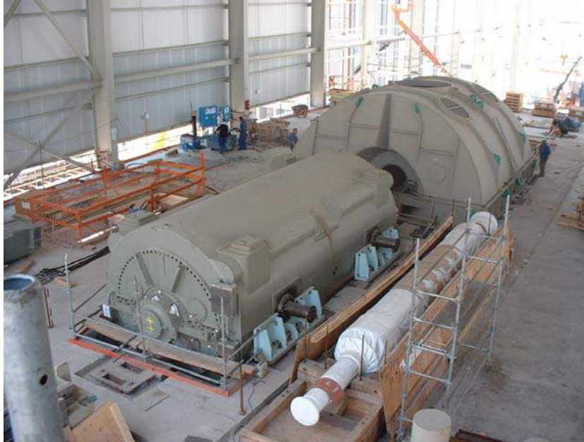
Turbogenerator 336MVA, 15.75 kV, 50Hz
