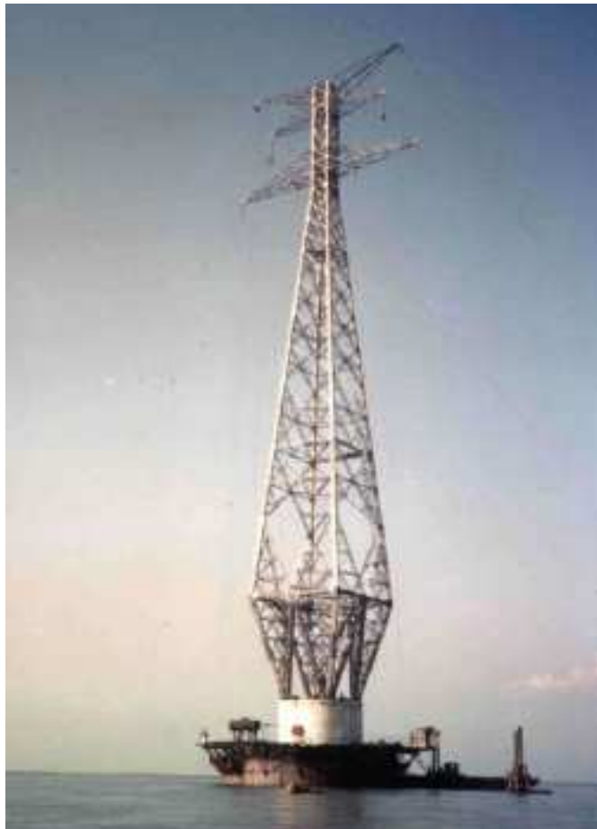
Figure 2: 230 kV Jamuna River crossing, Bangladesh
