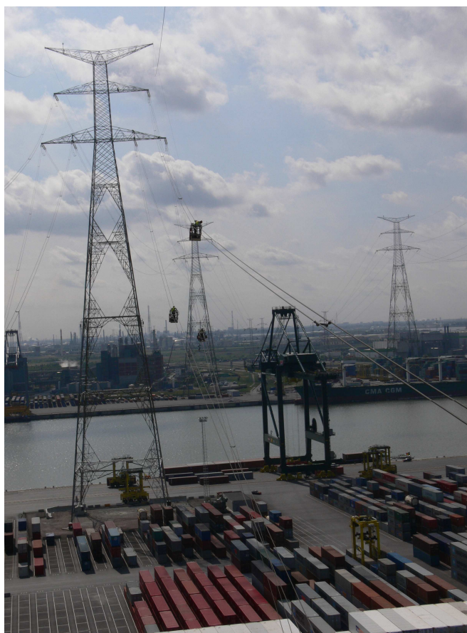
Figure 10: 380 kV "Deurganckdock Crossing": Doel, Antwerp, Belgium
