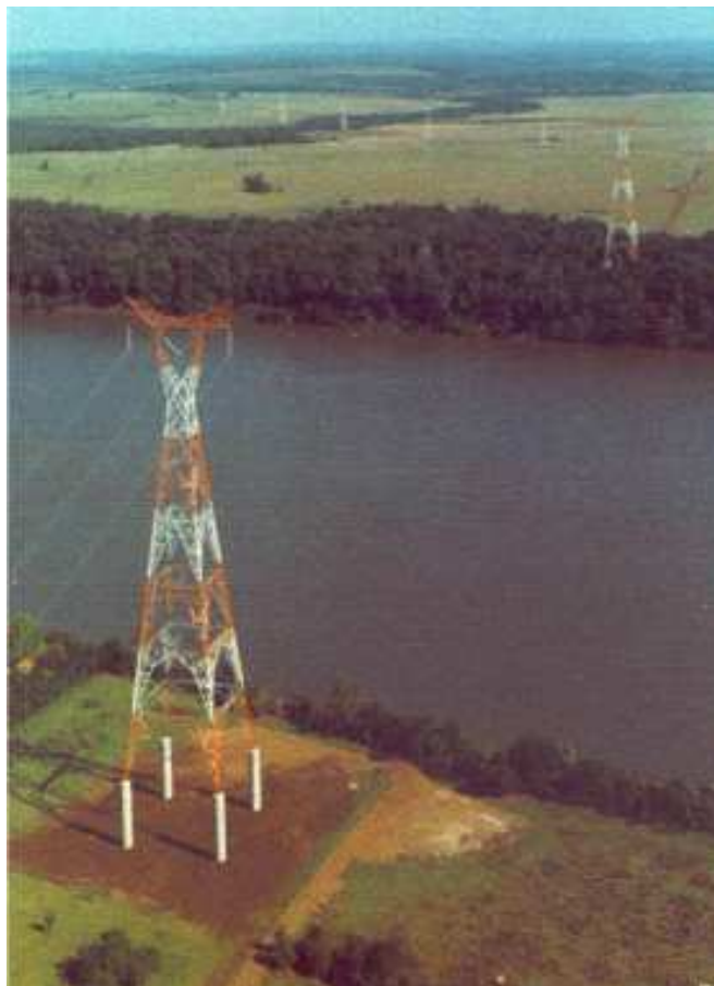
Figure 9: 500kV Uruguay River Crossing: Crossing with elevated foundations
