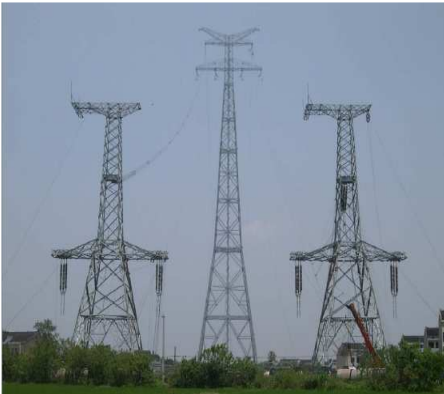
Figure 5: 500kV Jiangyin Yangtze River Crossing. In the foreground the anchor towers, one for each circuit. In the background one 346.5m tall suspension tower.
