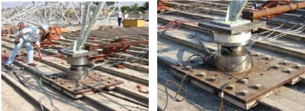
Figure 7: Device designed for application of displacements on tower
