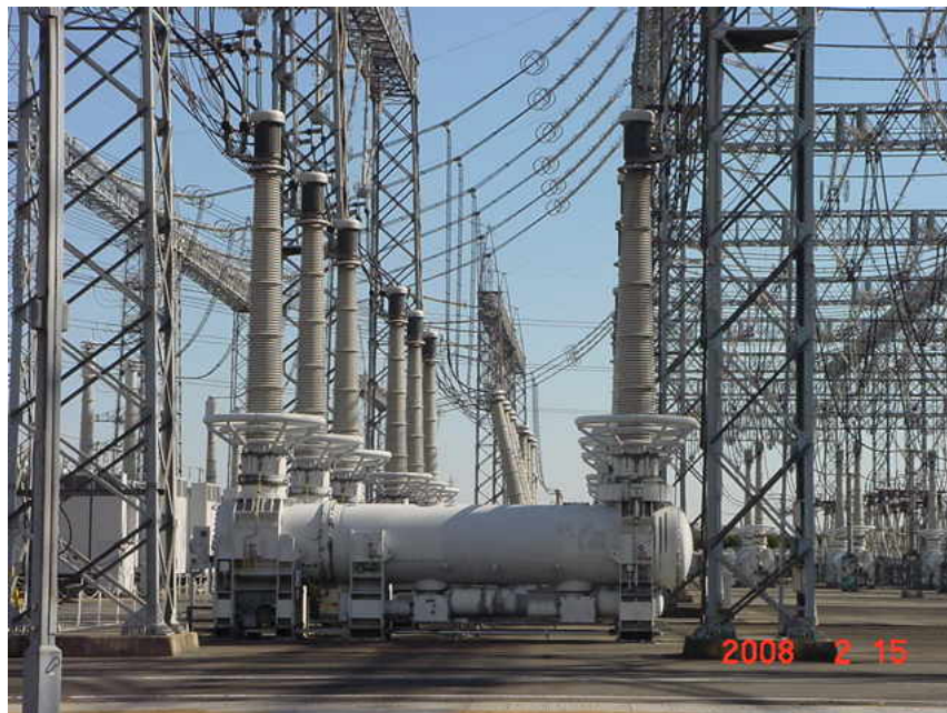
Partial replacement 1 break GCB from 4-break GCB
