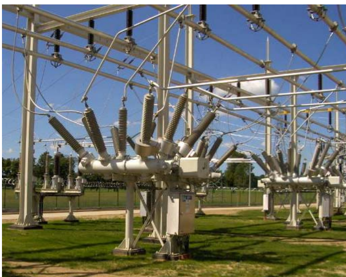
Fig 6: part of Hybrid IS Bay
