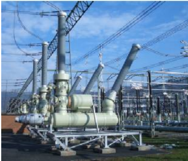
Fig 7: part of Hybrid IS
