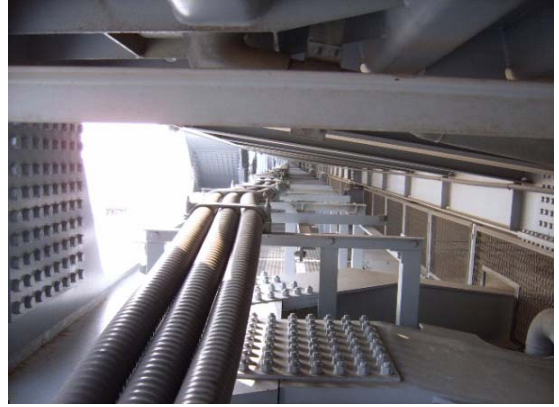
Figure 8.11.1 154kV power cables installed on Yeong-Jong bridge showing the snaking arrangement for bridge movement, joint installation and cable snaking in general.
