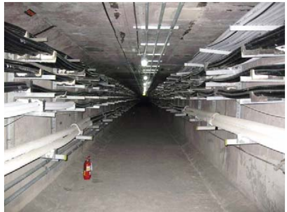
Figure 8.11.2 Examples of power cables and other services installed in Yeouido Shared Tunnel
