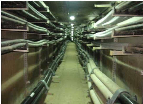
Figure 8.11.3 Examples of power cables installed in Jungdong Shared Tunnel
