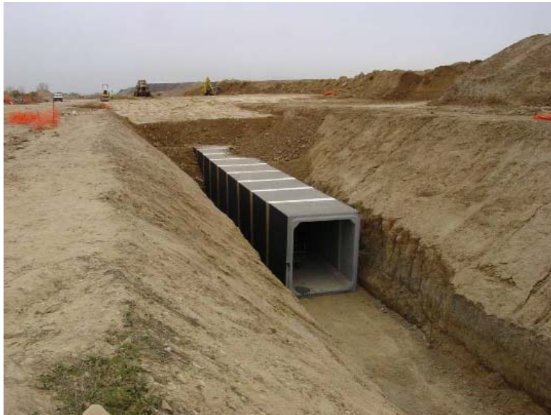
Figure 2.1.2 Cut and cover tunnel under construction in Madrid (Barajas)
