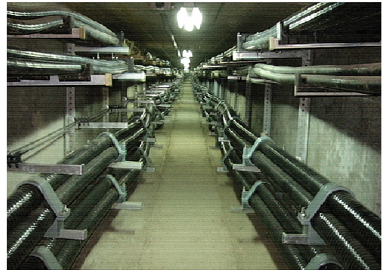
Figure 8.11.3 Examples of power cables installed in Jungdong Shared Tunnel
