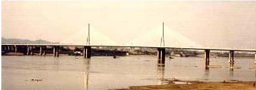
Figure 8.4.1 A general view of the Changsha River Bridge
