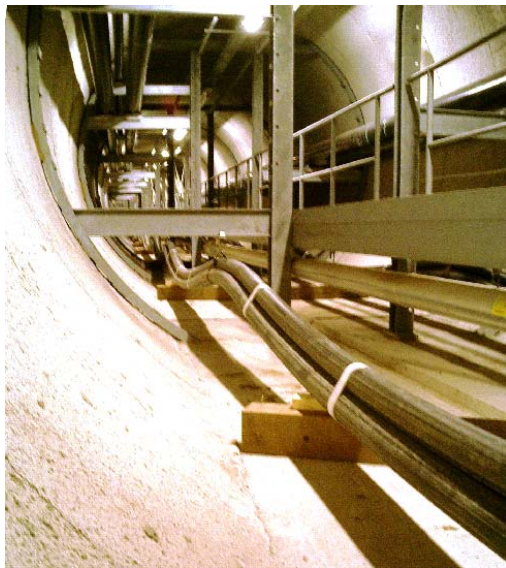
Figure 5.4 A multi purpose tunnel with two 150 kV power cable circuits and multiple pipes for gases and liquids (water, chemicals).
