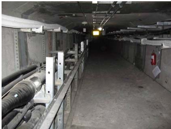
Figure 8.11.2 Examples of power cables and other services installed in Yeouido Shared Tunnel
