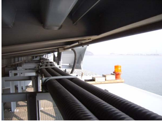
Figure 8.11.1 154kV power cables installed on Yeong-Jong bridge showing the snaking arrangement for bridge movement, joint installation and cable snaking in general.
