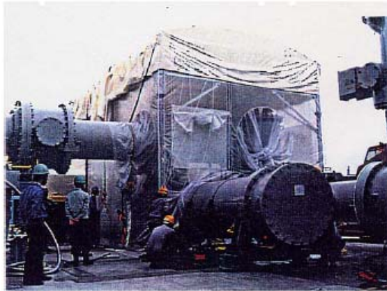
Fig. 92 all-weather dust-proof housing for GIS erection
