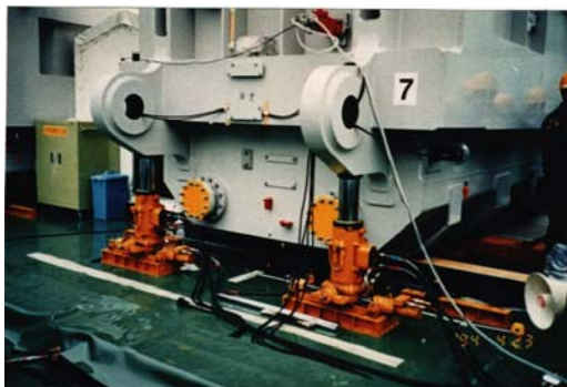
Fig. 93 Unit tank docking procedure for core-form UHV transformer
