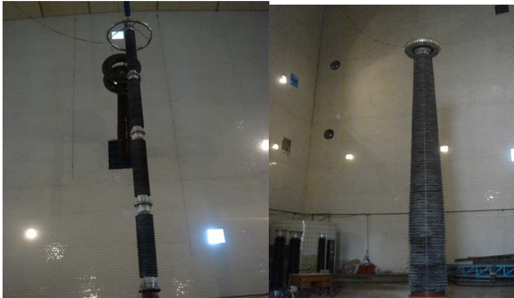
Fig. 13 The test arrangement of post insulator and hollow bushing shell
