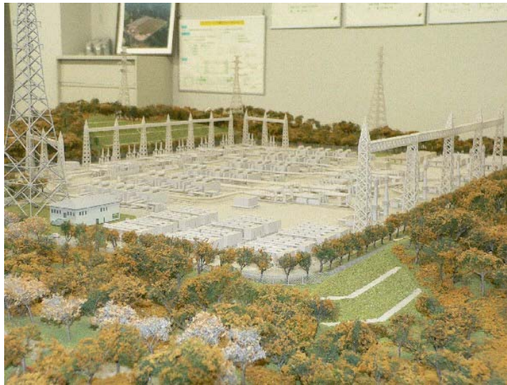
Fig. 1 UHV substation model to check the harmonization with the landscape (TEPCO 1100kV GIS)
