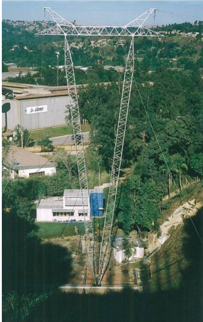
Figure 4 – Test arrangements - 500 kV TL Guyed Tower
