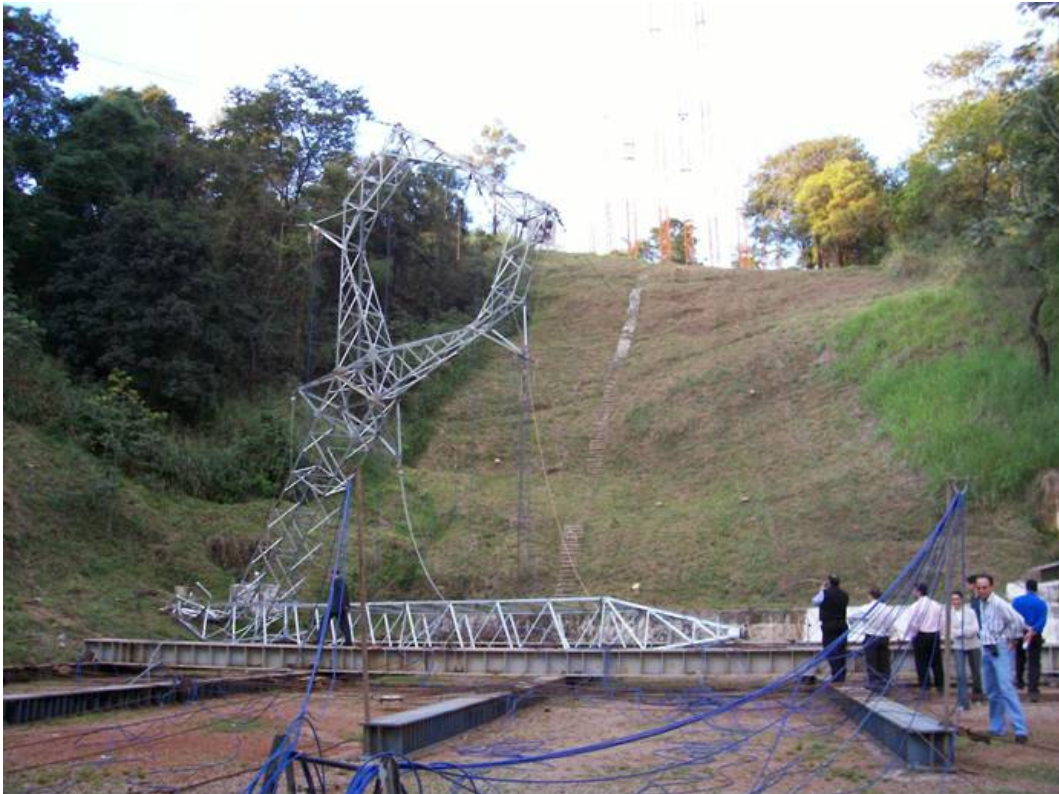
Figure 3 – Destructive test –230 kV TL Guyed tower
