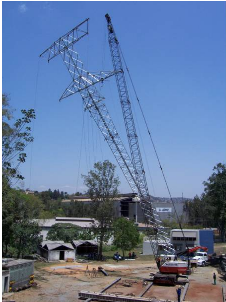
Figure 1 – Tower erection – 230 kV Double circuit guyed tower
