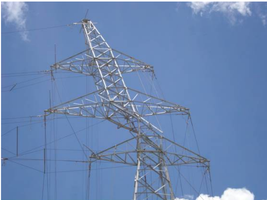
Figure 2 – Destructive test – 230 kV Double Circuit tower
