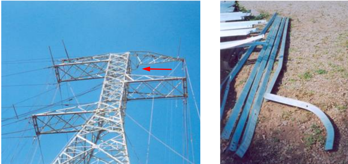
Figure 11 – Failure at 75 % loading
