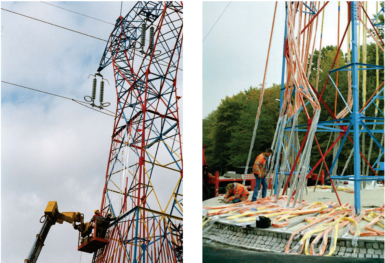
Figure 60 - Erection of the artwork of "Source"
