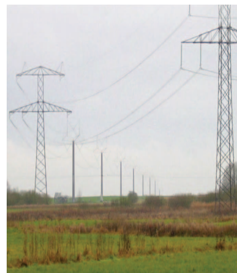
Figure 22 - Transition from Donau- to design-towers
