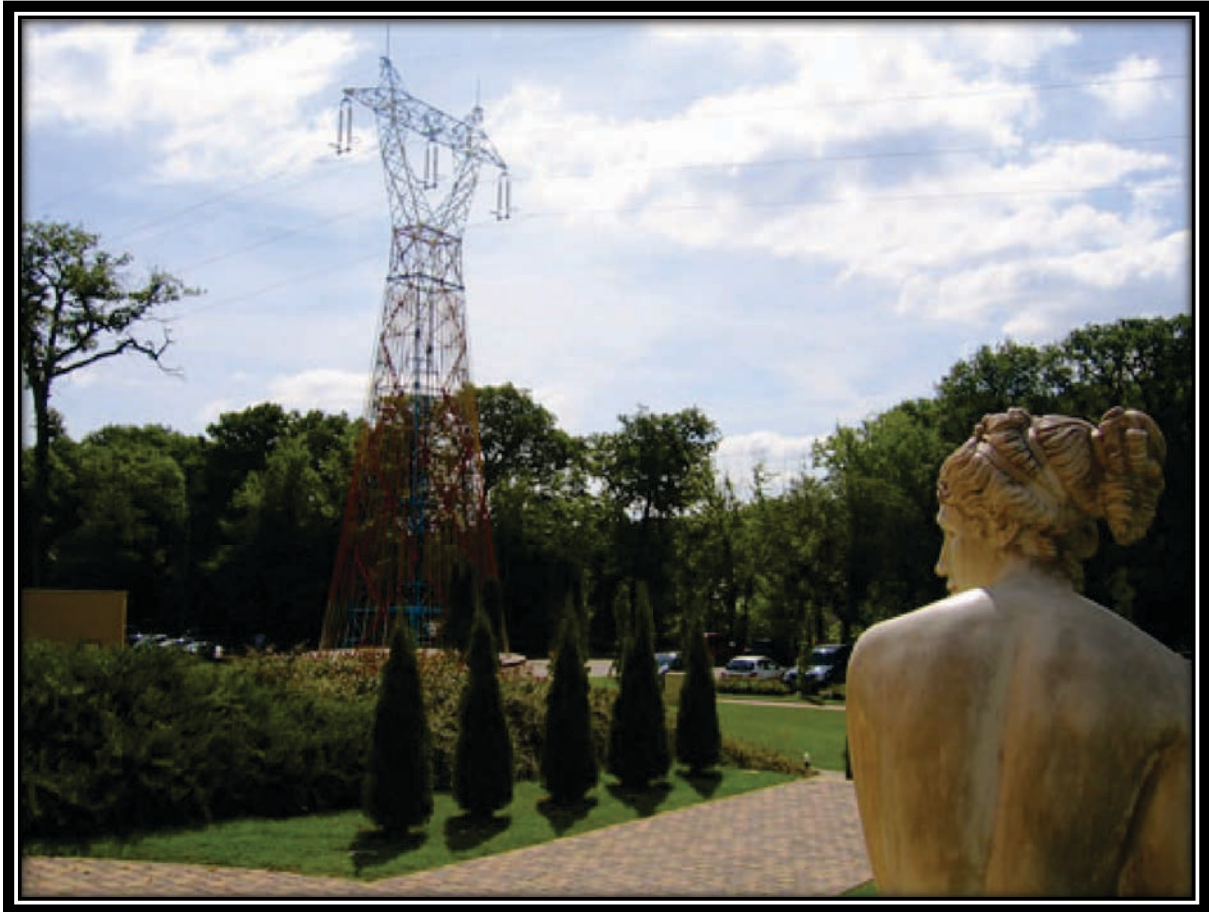
Figure 66 - "Source Flame" – Pylon n° 13
