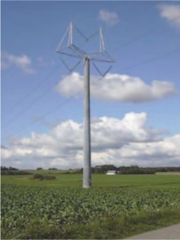
Figure 25 - Suspension V-string
