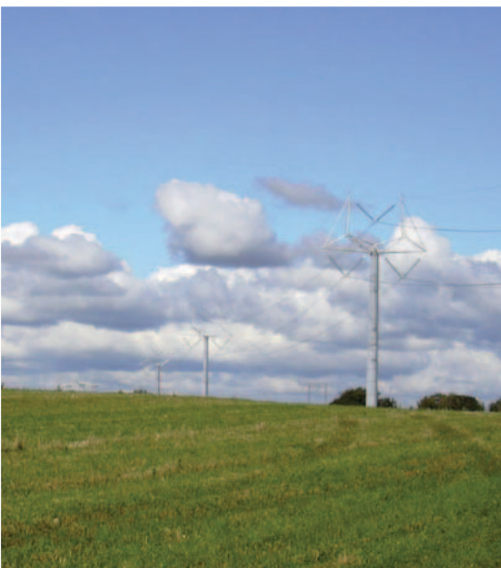
Figure 24 - Shafts in the landscape
