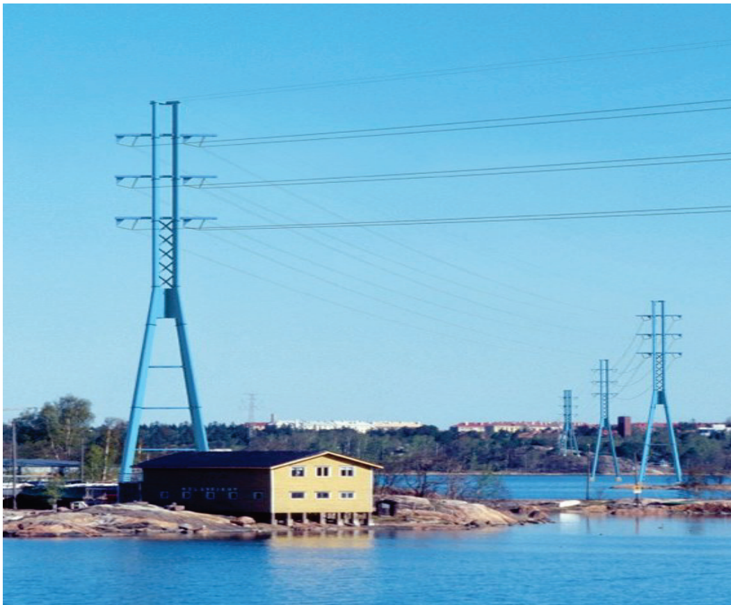
Figure 31 - A photo montage of the transmission line
