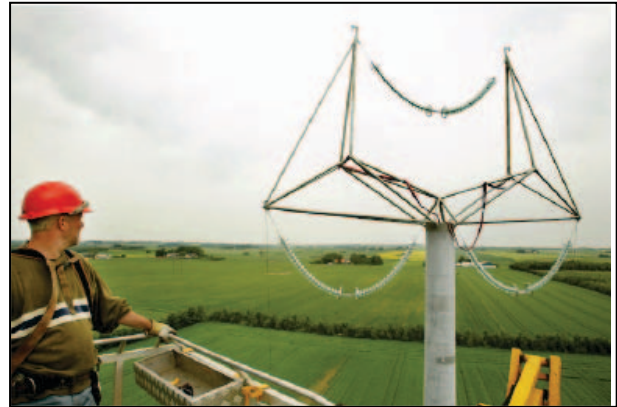
Figure 23 - The lattice top
