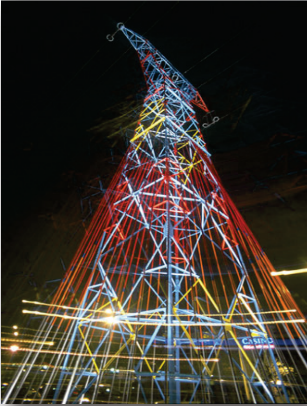
Figure 64 - "Source Energy" – Pylon n° 12
