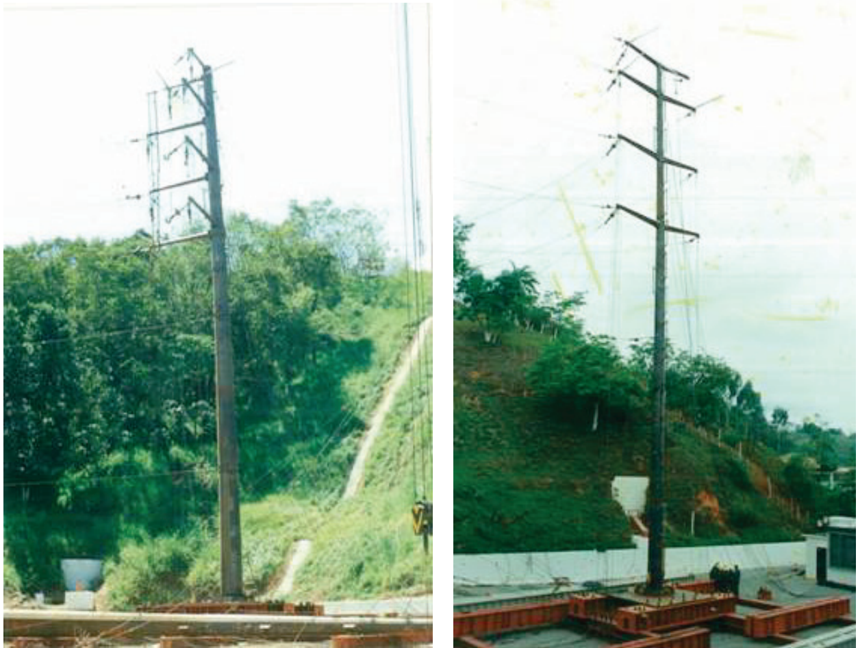
Figure 9 - Pole deflections during Tests
