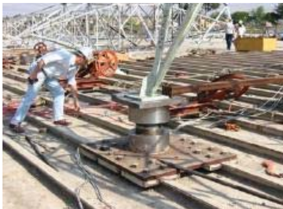
Figure 7: Device designed for foundation displacements
