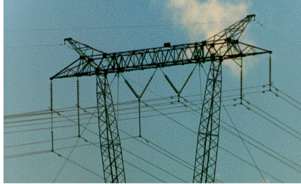
Figure 17: Experimental HSIL line in Brazil: the right circuit is conventional. The bundle of the left circuit has been expanded as to increase the surge impedance loading.
