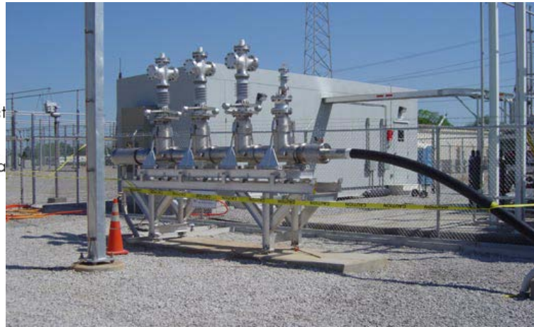
Fig. 4.9: Termination of Triax cable
