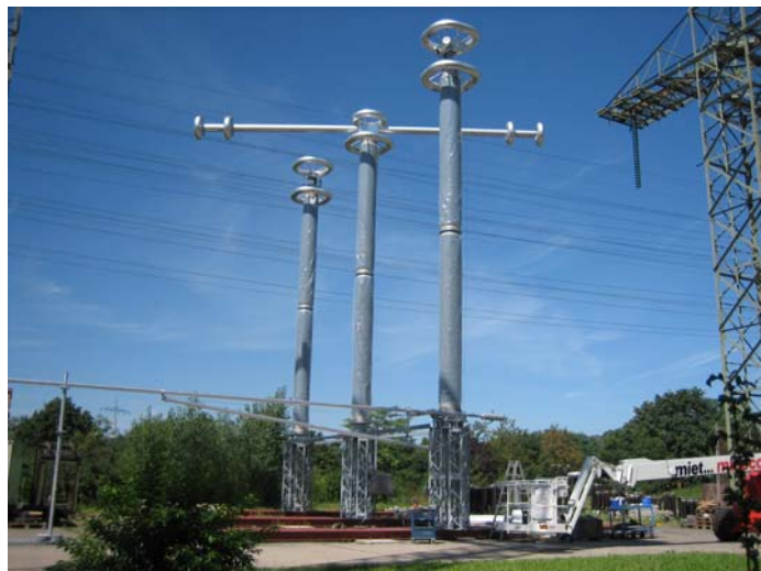
Figure 3.8 DC Double break isolator (Courtesy Siemens)
