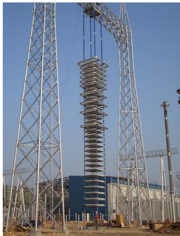
Figure 3.10-DC filter capacitor under installation (Courtesy Siemens)
