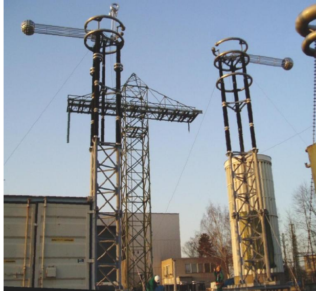
Figure 3.7 DC single break isolator (Courtesy Areva)
